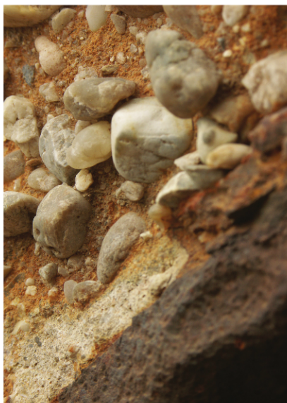
Fig. 1: Contaminated concrete remaining on surface following surface preparation. All photos courtesy of the author.
