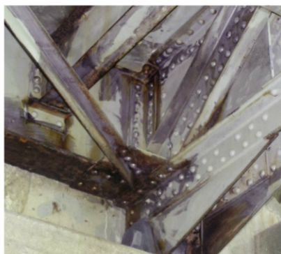
Fig. 1: Failed coating beneath a leaking joint. All photos and figures courtesy of Kentucky Transportation Center, University of Kentucky unless otherwise specified.
