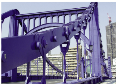
Fig. 7: Certain bridge components such as seams, edges, bolts and rivets still present coating and life cycle challenges, even for FEVE-based coatings.
