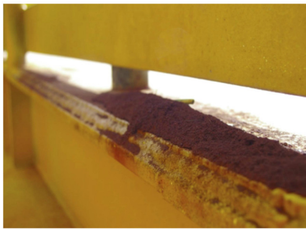
These two prints show examples of prodigious amounts of grinder dust on an offshore gas platform resulting from hotwork after the paint system was applied.
