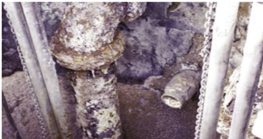
Fig. 4: In order to write a coating specification properly, the specifier must first be able to recognize microbially induced corrosion (MIC), such as on these lift station components.
