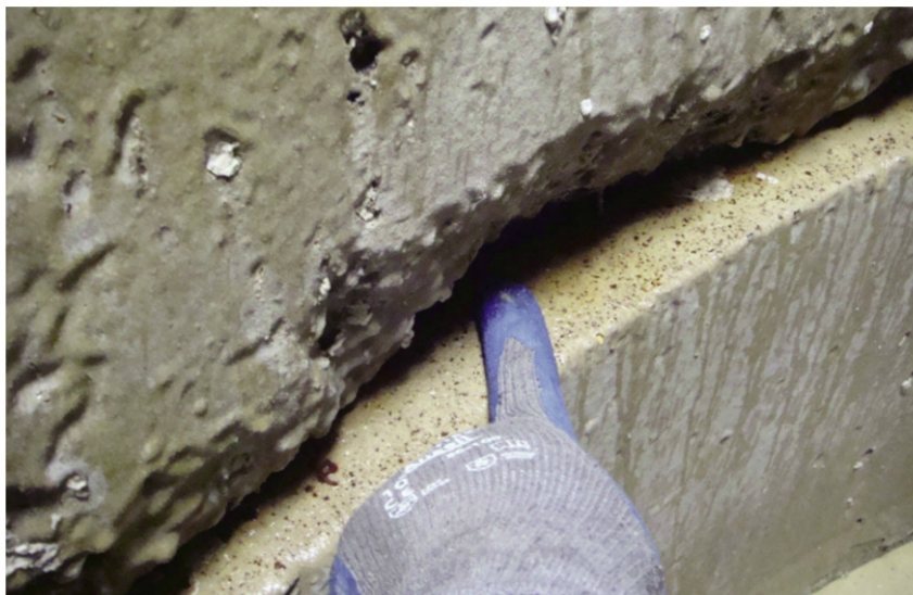
Fig. 7: This concrete joint in a wastewater holding tank should have been filled and sealed prior to coating application.
