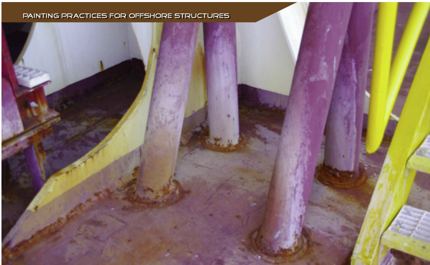
Here is an example of the inadequate preparation and painting of hotwork zones around circular hollow section columns where they were welded to the tank deck.
