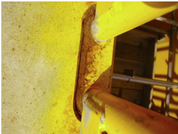
These two prints show examples of prodigious amounts of grinder dust on an offshore gas platform resulting from hotwork after the paint system was applied.
