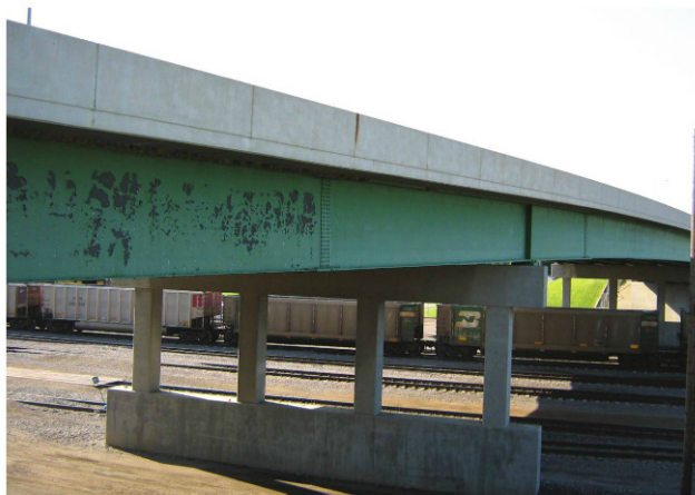
Fig. 1: Pictured here is a bridge where only one girder had thick, uncured zinc. Note the significant failures. The other girders were cured and had no failures. Photos courtesy of KTA-Tator, Inc.
