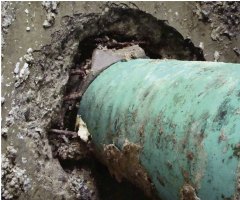
Fig. 3: Pipe penetrations that are not filled and sealed properly prior to immersion can be more vulnerable to corrosion.
