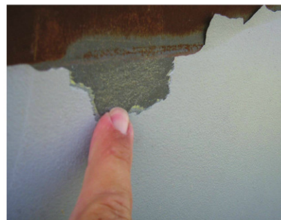
Fig. 2: This photo shows an area where the IOZ had been exposed for a couple weeks. When the topcoats were pulled away separation occurred within the zinc layer, with zinc on the back of the delamination and left on the bridge.
