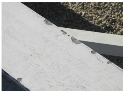
Fig. 3: Excessive impact damage on a light rail line that occurred during erection is visible in this image.
