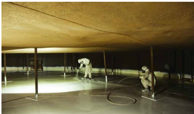
Fig. 4: Spray application of the gel coat in a spray-applied, chopped-strand system Photo courtesy of Švykai UAB
