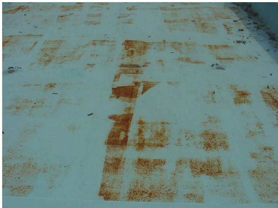
Fig. 1: Widespread rusting over a swimming pool bottom due to high surface profile and/or low coating thickness. Photos courtesy of KTA-Tator, Inc.
