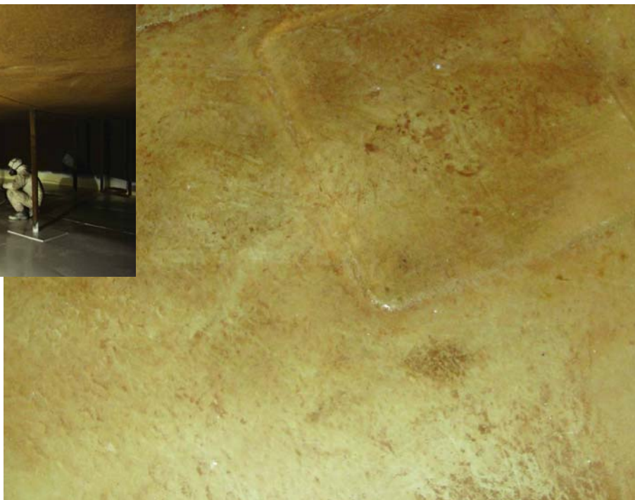
Fig. 5: After 15 years in service, this spray-applied, chopped-strand system shows no defects during inspection
