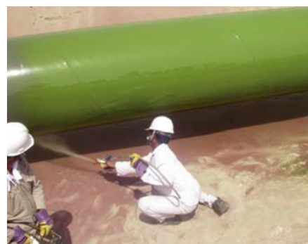
Fig. 5: Application of test coating in the Middle East
