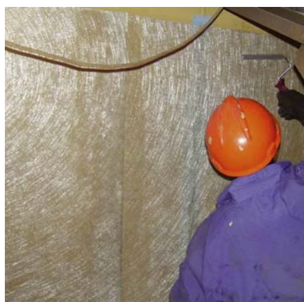
Fig. 2: Rib-rolling the reinforcement mat in a hand-lay system to remove entrapped air and ensure good wetting out
