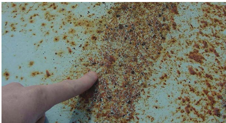
Fig. 2: Closer view of pinpoint rusting on pool bottom; more concentrated areas of rust typically had a higher surface profile.
