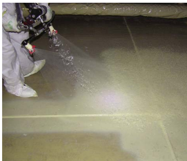
Fig. 3: Application of the spray-applied, chopped-strand system
