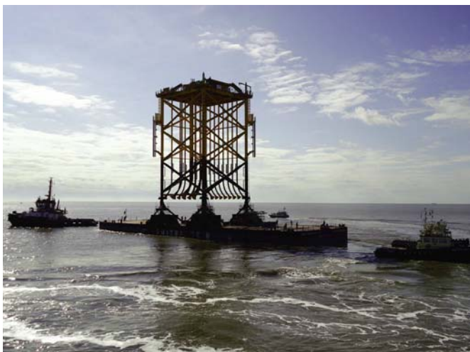
(Above and below): Finished jackets were loaded from the facility onto barges and then shipped out for placement at the Thornton Bank.
