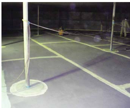
Fig. 1: Caulking and stripe coating completed
