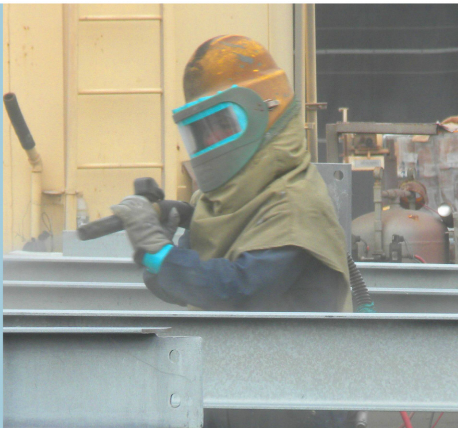
This blaster is using medium-grade garnet abrasive to obtain a Commercial Blast Cleaned surface (SSPC-SP 6) and a 2-to-3-mil anchor profile.
