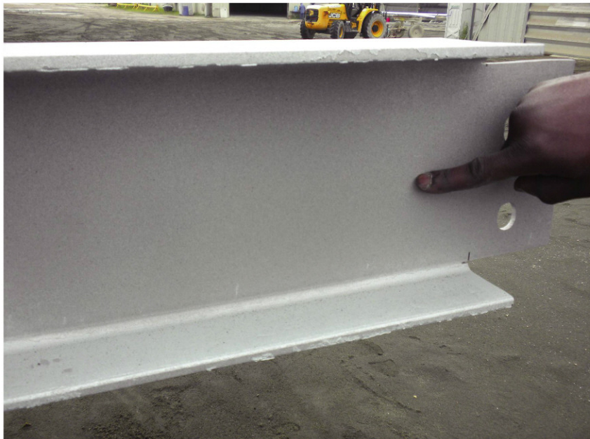
Beam end area has been blasted to a "Near White Metal" finish (SSPC-SP 10).
