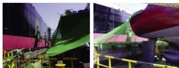
Fig. 2: Installation of the protection net
