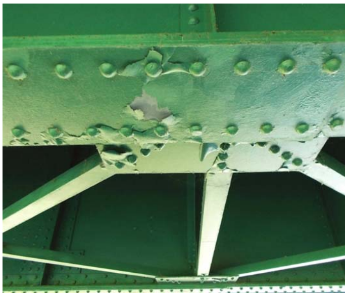
Figs. 6 and 7: Coating System K, the zinc-rich moisture-cured urethane and polyaspartic urethane showed rust, peeling and cohesion failure on approximately 10 percent of the total surface area.
