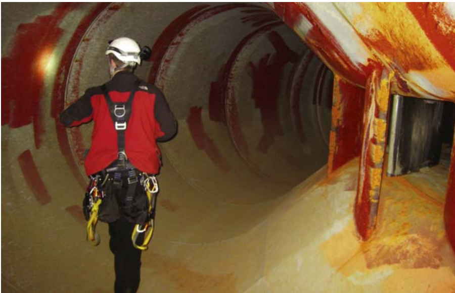
Fig. 5: Scroll case, stay vanes, and wicket gates with previous spot repairs
