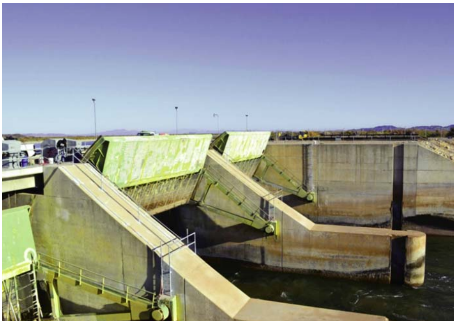
Fig. 3: Reclamation transferred works, which includes a radial gate structure with fluctuating immersion exposure
