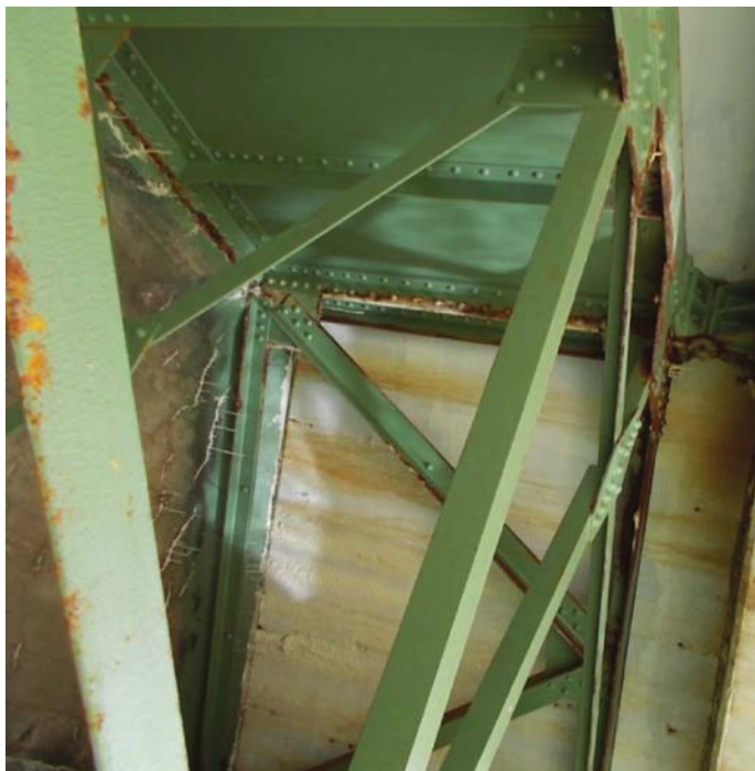
Figs. 4 and 5: Coating System J, the elastomeric acrylic, showed blistering, peeling and corrosion on approximately 20 percent of the total surface area.
