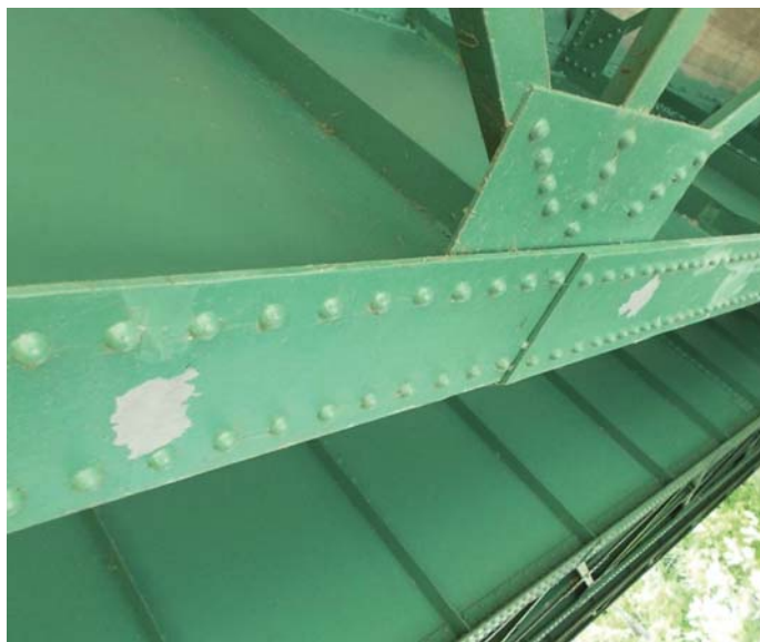
Figs. 6 and 7: Coating System K, the zinc-rich moisture-cured urethane and polyaspartic urethane showed rust, peeling and cohesion failure on approximately 10 percent of the total surface area.
