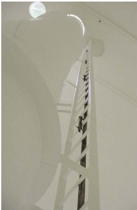
The tank's interior immersion surfaces, including ladders and other appurtenances, received 100% reconditioning in 2006.
