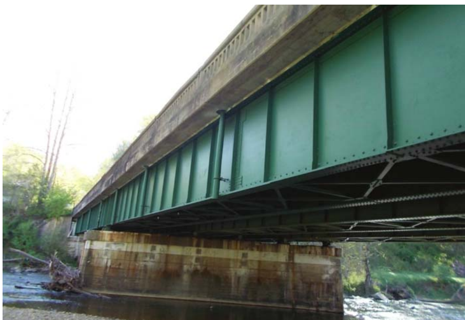
Figs. 1 and 2: Bridge No. 0700300 in Maryland was selected because it provided three coating surfaces independent of one another, is in a humid environment, and suffers from leaky joints and an old concrete deck with high salt concentrations. Winter salt spray can penetrate cracks in concrete bridge decks. When the deck dries, the salt remains.
