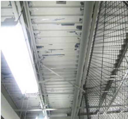
Fig. 3: Areas of coating delamination where Coating B was applied
