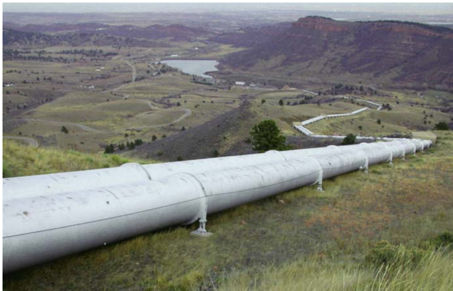
Fig. 2: The Flatiron Penstocks (Loveland, Colo.) feature a long pipe span and a rugged slope at a 15-degree incline.
