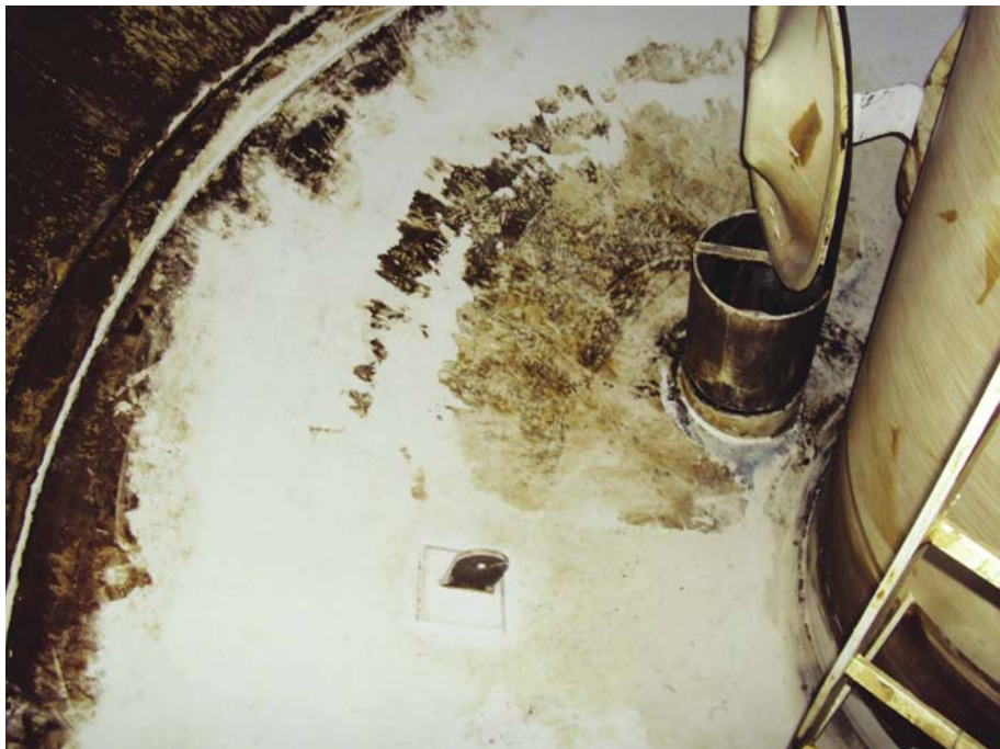
By 2010, tank immersion surfaces were exhibiting staining and sediment build-up, requiring power washing and sediment removal.
