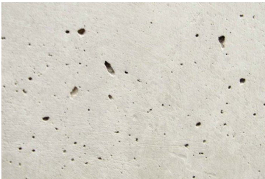
Fig. 5: Typical bug holes on formed concrete
