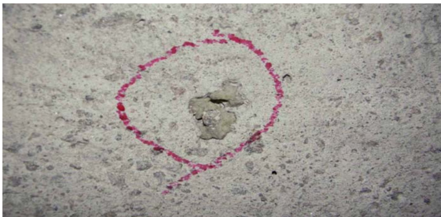
Fig. 6: Residual lining material (substrate was prepared by UHPWJ followed by abrasive blasting)
