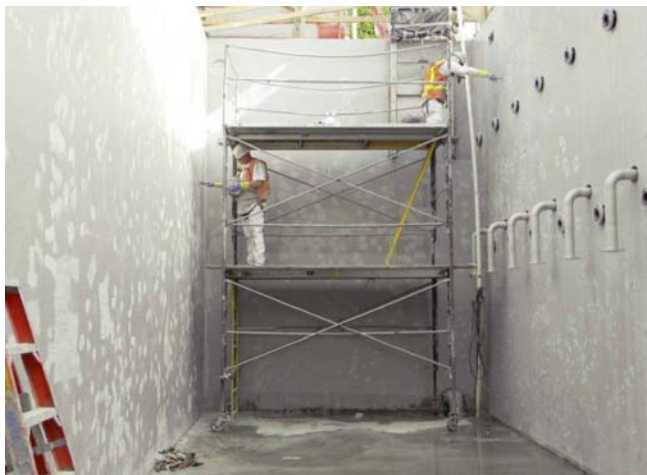
Fig. 10: Repairing holidays. Most specifications do not set a limit for the maximum number of holidays allowed, either for the entire structure or expressed as a holiday to substrate area ratio.
