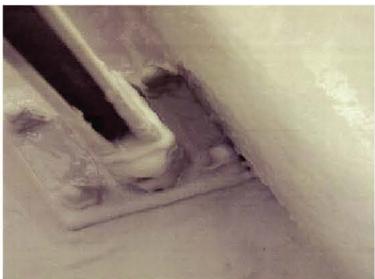
Fig. 4: Close-up of polyurea-coated unistrut design detail and geotextile membrane
