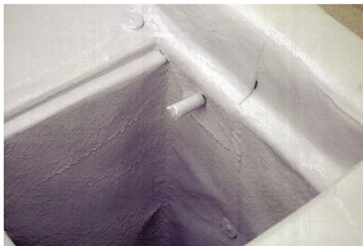
Fig. 5: Installation of liner in sump
