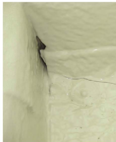
Fig. 8: Rupture in lining caused by fabric "tenting"
