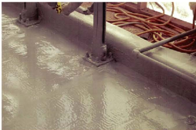
Fig. 3: Polyurea-coated unistrut design detail
