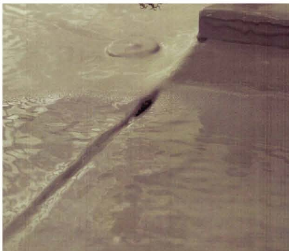
Fig. 7: "Bird mouths" at geotextile seams
