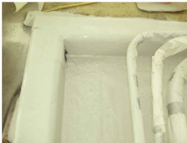
Fig. 2: The polyurea/geotextile loose liner system contoured to surfaces to which it was applied.
