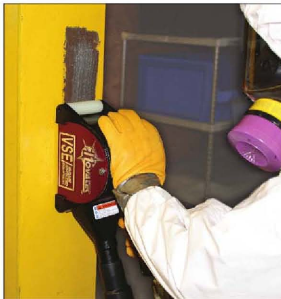
Vacuum-shrouded roto peening prep tool used on a vertical surface. Courtesy of Novatek Corp.
