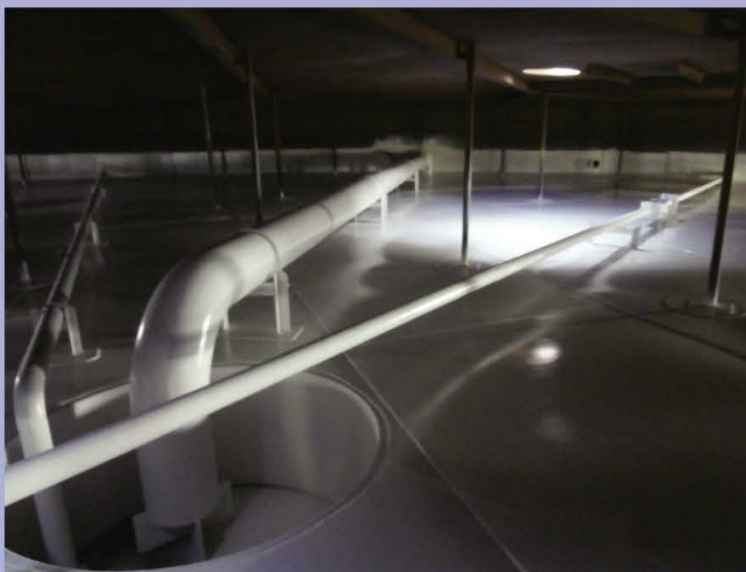
Pictured is the newly finished interior of a crude oil storage tank where a routine inspection revealed a significantly degraded floor. The owner did not have time to wait for standard linings to cure, so a fast return to service lining was specified. Photo courtesy of Sherwin-Williams.
