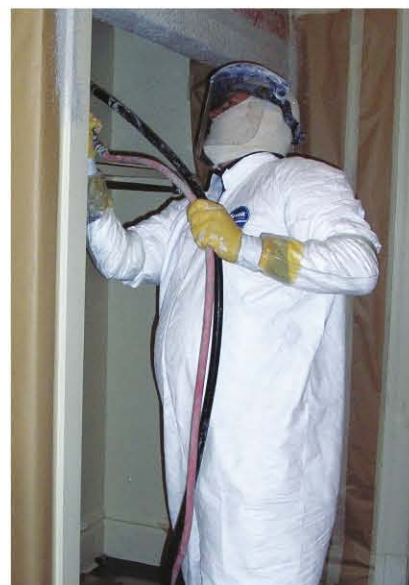
Worker protection is essential when using chemical strippers to remove coatings. Photos courtesy of Dumond Chemicals, Inc.
