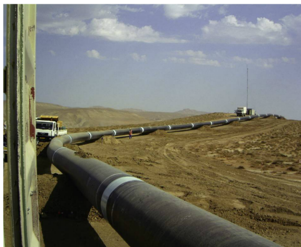
Fig. 1: Onshore field joint coating
