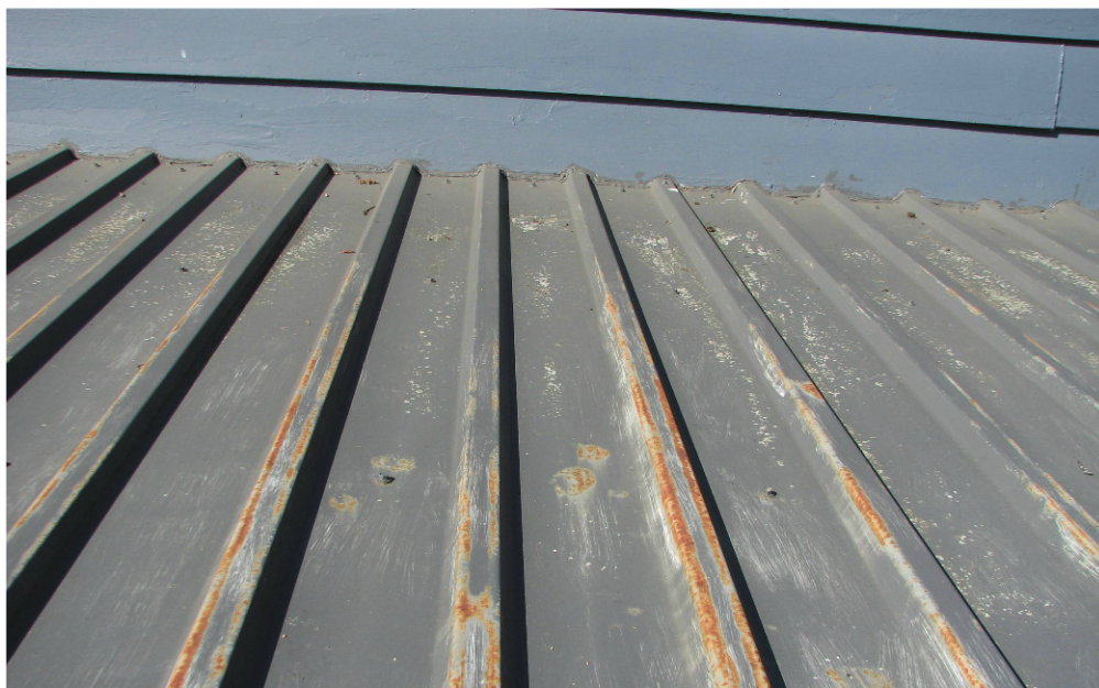
Fig. 3: The coating used on this metal roof had poor UV resistance and degraded significantly.
