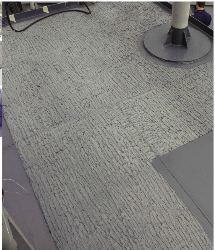
Fig. 2: This image depicts a color-faded and degraded epoxy non-skid on the deck surface of a ship less than six months after installation.
