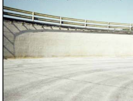
Polyurethane lining in paper mill wastewater treatment clarifier 21 (concrete substrate)
