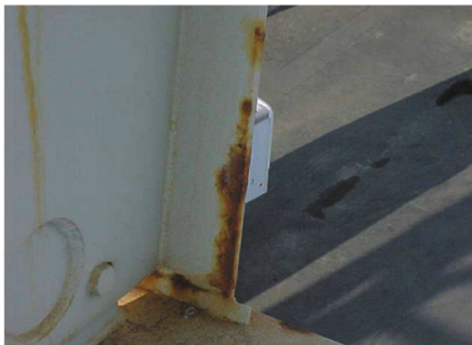
Edge failure on stiffener that was not stripe coated
