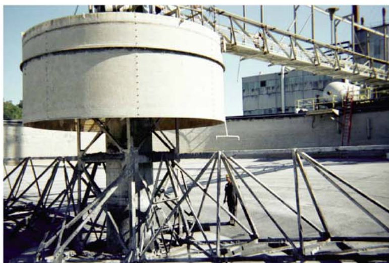
Polyurethane lining in paper mill wastewater treatment clarifier 21 (steel substrate)
