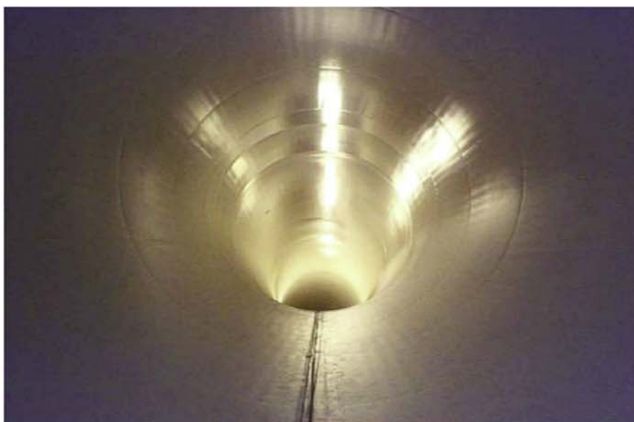
Polyurethane hybrid lining on steel internals of penstock 8
