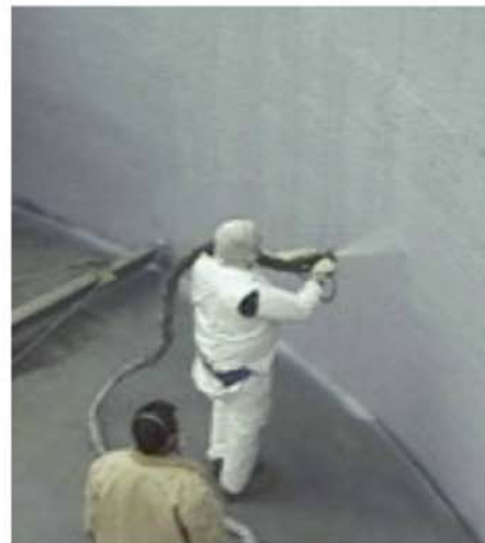
Polyurea lining in wastewater treatment clarifier 26 (concrete substrate)
