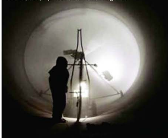
Polyurethane hybrid lining 8 in a penstock (steel substrate; robotic, self-propelled automatic blasting unit)
