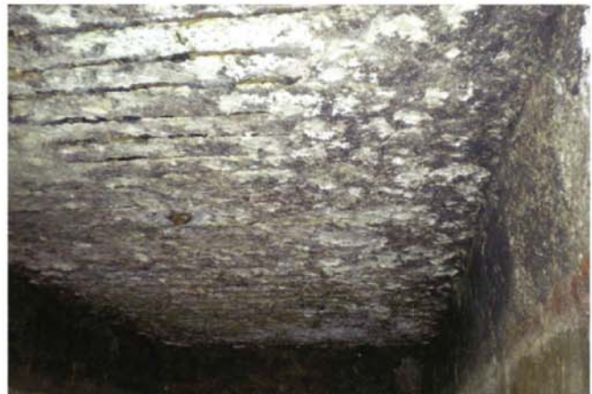
Fig. 2: Severe concrete corrosion in the ceiling of a regional wet well structure
