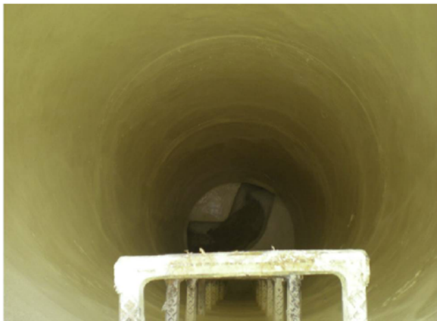
Fig. 7: Flexible polyurethane elastomer lining in a sanitary sewer collection system Courtesy of Carolina Management Team
