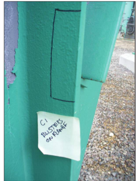
Fig. 3: Blisters formed in the polyurethane finish coat on a flange
