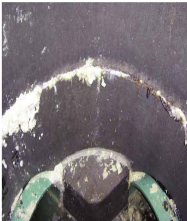
Fig. 11: Stopping a high-volume leak with hydrophillic polyurethane chemical grouts Courtesy of DeNeef Construction Chemicals
