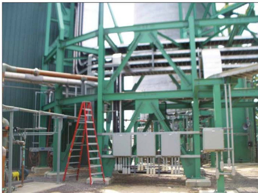
Fig. 1: Sections of newly-coated steel members at a coal-fired power plant displayed blistering and other signs of coating failure. Photos courtesy of James D. Machen, KTA-Tator, Inc.
