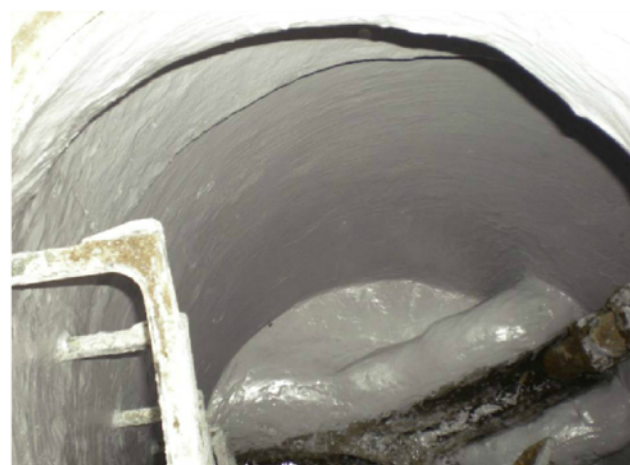
Fig. 6: Epoxy mortar lining in a sanitary sewer manhole Courtesy of Carolina Management Team
