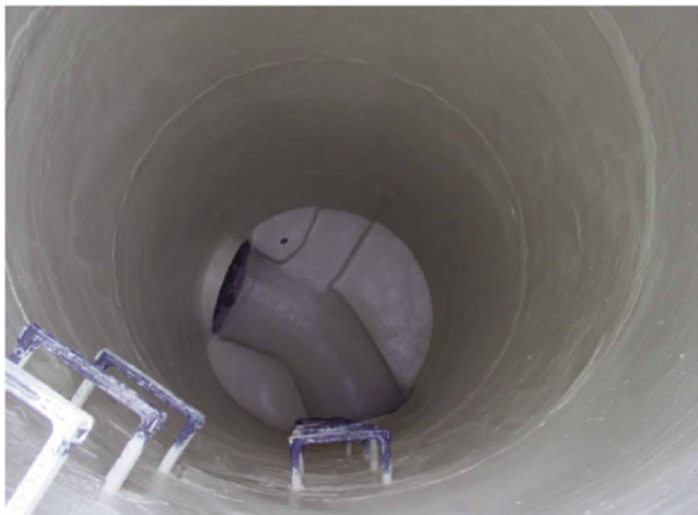
Fig. 8: Flexible polyurethane elastomer lining system in a sanitary sewer manhole Courtesy of The Sherwin-Williams Company
