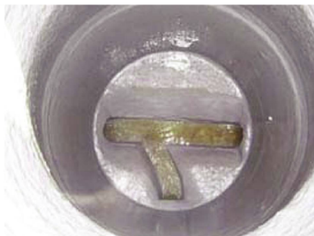
Fig. 9: Polyurea lining system in a sanitary sewer manhole Courtesy of PCT 360
