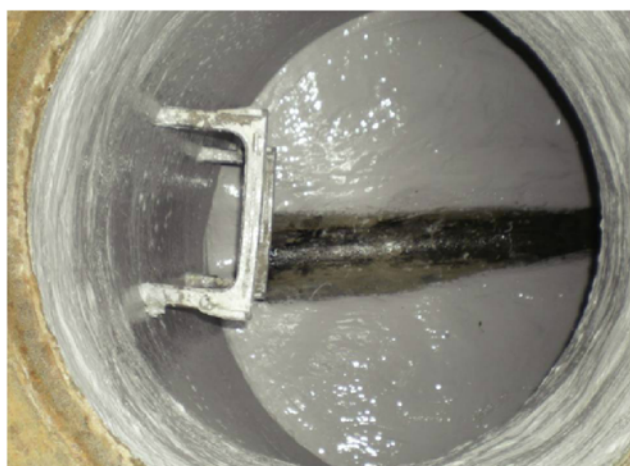
Fig. 5: High-build epoxy lining system in a sanitary sewer manhole Courtesy of Carolina Management Team
