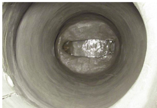
Fig. 4: Cementitious rehabilitation of a sanitary sewer manhole Courtesy of Southern Trenchless Technologies
