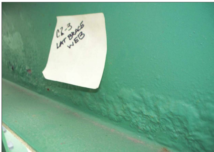
Fig. 4: Blisters in the polyurethane finish coat on a lateral brace web
