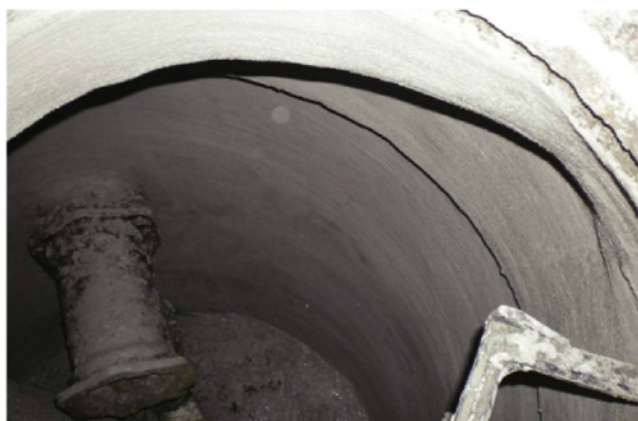
Fig. 3: Cementitious rehabilitation of a sanitary sewer structure Courtesy of Carolina Management Team
