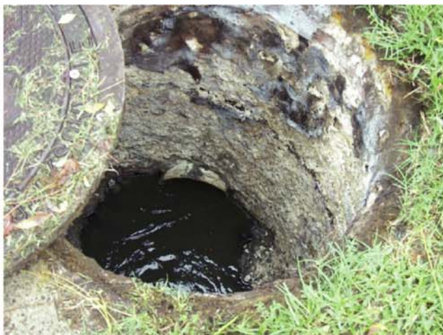
Fig. 1: Severely corroded sanitary sewer manhole Courtesy of The Sherwin-Williams Company
