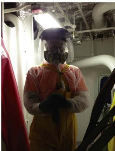
Worker preparing to enter confined space to perform degassing and cleaning
