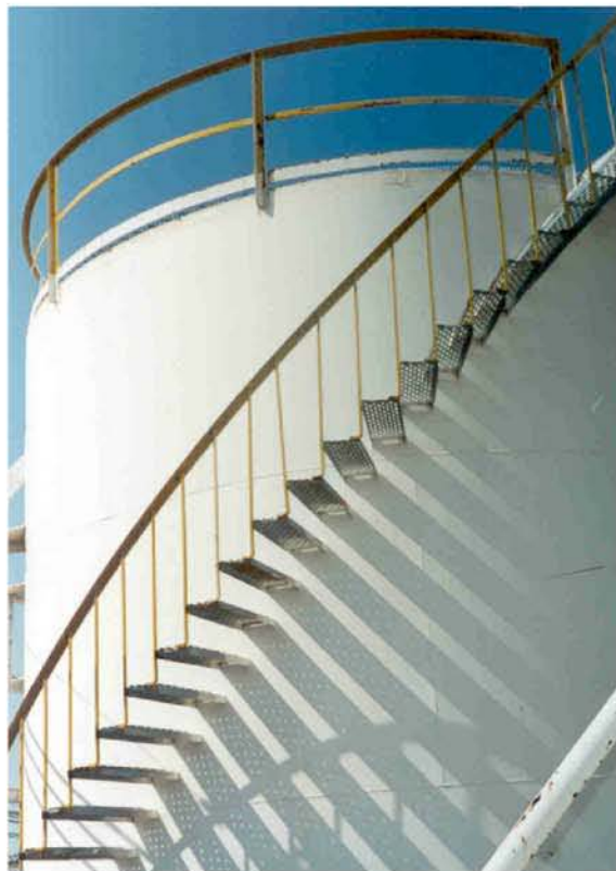
Fig. 4: A chemical storage tank located in a chemical plant in Philadelphia, PA. The tank was coated with a three-coat waterborne acrylic system in 1986. The tank is shown here after 15 years of exposure.
