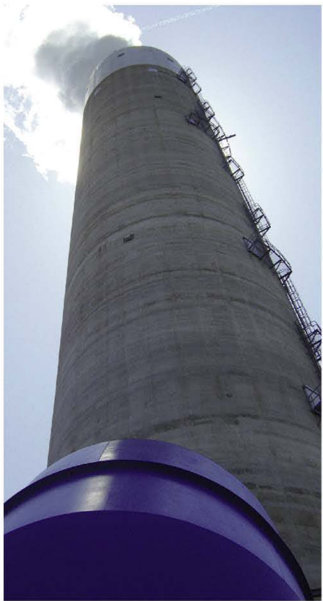
Outlet duct and chimney. Linings must protect against saturated environments that have high permeation potential, especially when subjected to cold wall effects.
