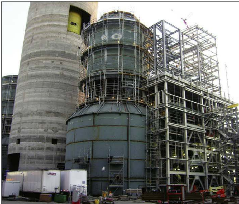
Absorber towers offer many lining challenges in regard to temperature, low pH, high chlorides, and abrasion from direct impingement and agitation.
