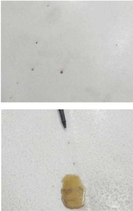
Fig. 5a (top) shows holes in the floor where the amber residue was wiped up and Fig. 5b (bottom) where the amber material was still present on the surface.
