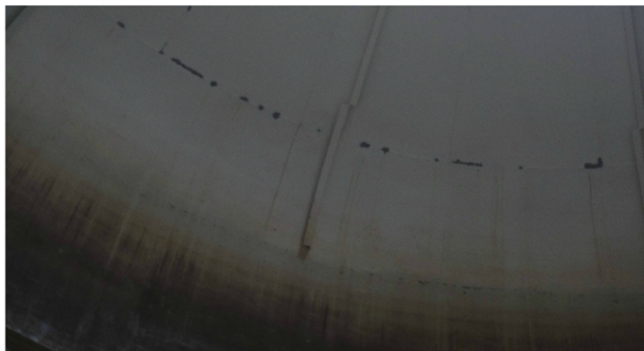
Fig. 11: 2011—Preparation of spot repair areas for two-coat epoxy
