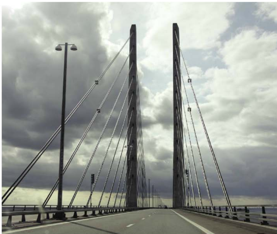
Fig. 2: The Øresund bridge, connecting Sweden and Denmark. The coating system (using a zinc-rich primer) has been designed to protect the bridge against corrosion for a period of at least 100 years.
