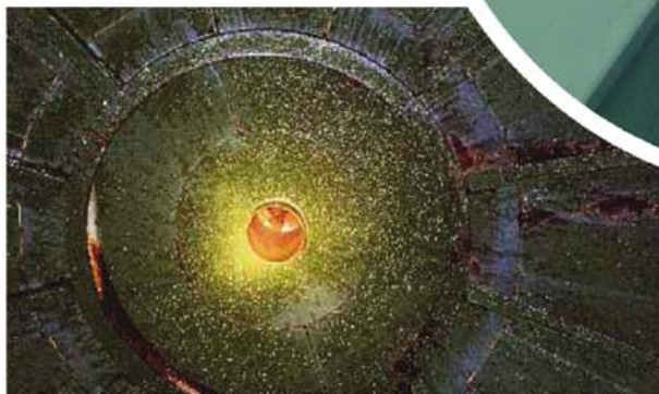
Fig. 1a (left): Condition of vapor area in interior of roof in 2001
