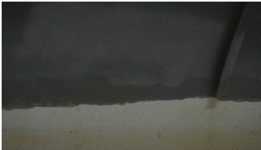
Fig. 9: 2011—Preparation of spot repair area of single-coat zinc
