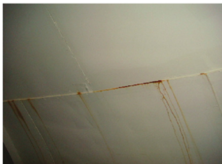
Fig. 4: 2009 inspection—minor failures in two-coat polyamide epoxy
