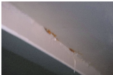
Fig. 7: 2011—Example of area for spot repair of two-coat epoxy system
