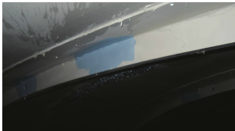
Fig. 12: 2011—Topcoated spot repair area with second coat of epoxy (used for repairs of two-coat epoxy and of three-coat zinc-epoxy-epoxy)
