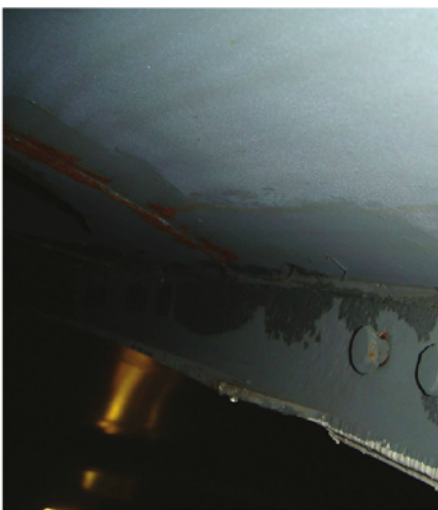
Fig. 5: 2009 inspection—spot failures of single-coat zinc, attributed to application error
