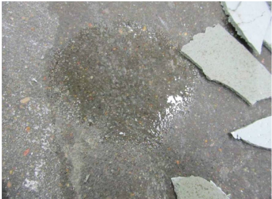
Fig. 7: Wet surface found below and intact blister.
