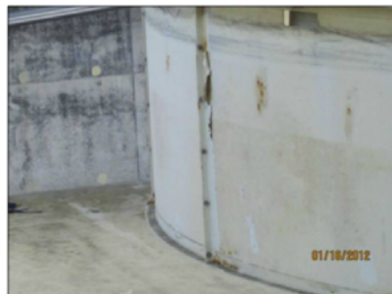
Fig. 7: Finish coat at bolted connection has delaminated on a clarifier.
