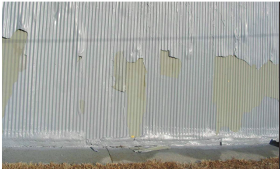
Figure 4: The extent of the coating system failure was dramatic when viewed on large portions of the building exterior walls.
