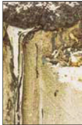
Fig. 3: Advanced sulfate attack of concrete exposed to high sulfate-bearing water
