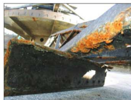
Fig. 4: Clarifier—immersed steel
