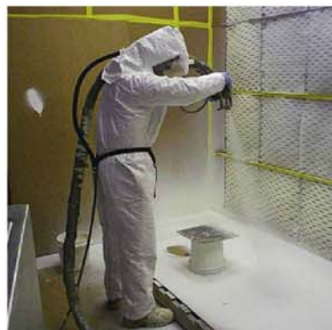
Fig. 6: Applicators must take appropriate measures to protect themselves while spraying polyurea.
