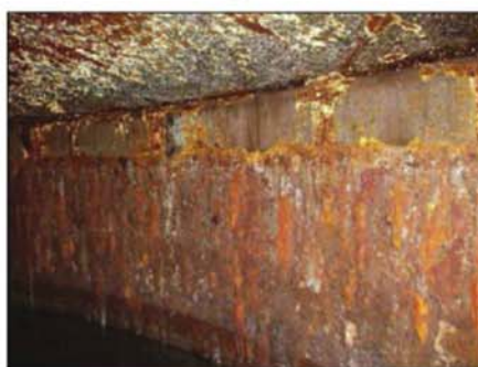
Fig. 1: Corroded steel water tank walls and roof above the water surface. Photos courtesy of the author.
