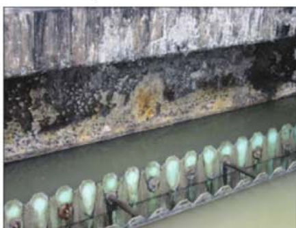
Fig. 2: Deteriorated interior atmospheric concrete in an enclosed primary sedimentation tank.
