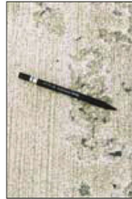
Fig. 4: Scaling of concrete deck in parking garage due to freeze-thaw cycle
