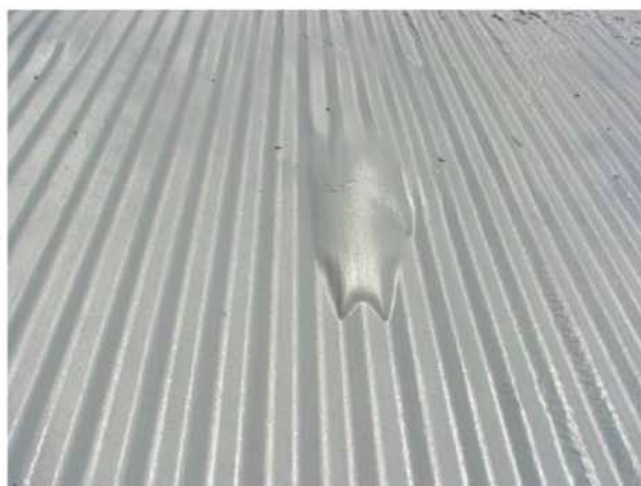
Figure 1: A large blister in the applied polyurea coating system. Photos courtesy of KTA-Tator, Inc.
