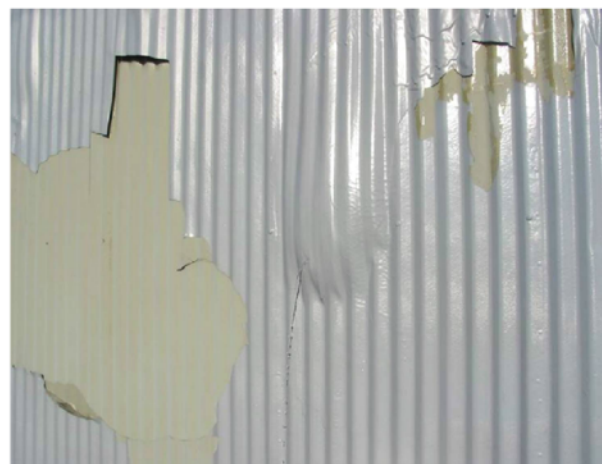
Figure 3: A large "sack" formed by the flexible polyurea coating leaked water when punctured near the base.
