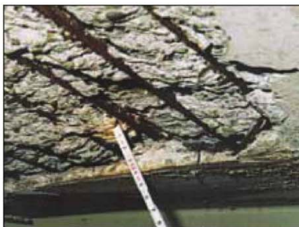
Fig. 1: Rebar corrosion of a bridge deck soffit Photos courtesy of Corrosion Probe, Inc.
