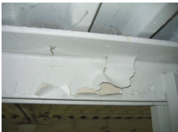
Fig. 2: Extreme delamination of the dry fall coating from the original alkyd on supporting steel
