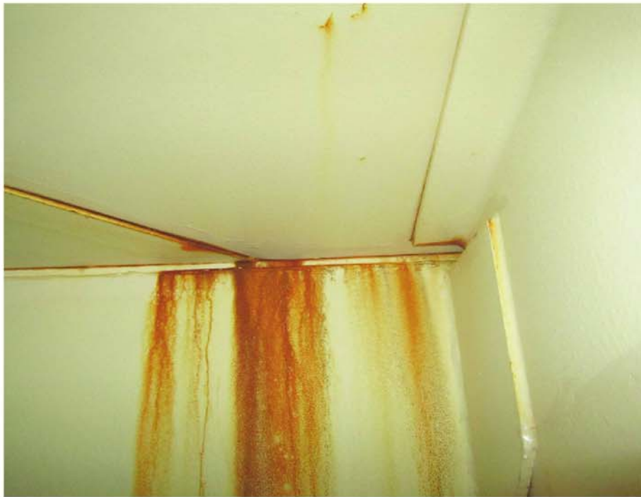
Fig. 9: Inside view of open side of lap weld. Rust is coming from the open side of the weld, which is difficult to protect with coatings.
