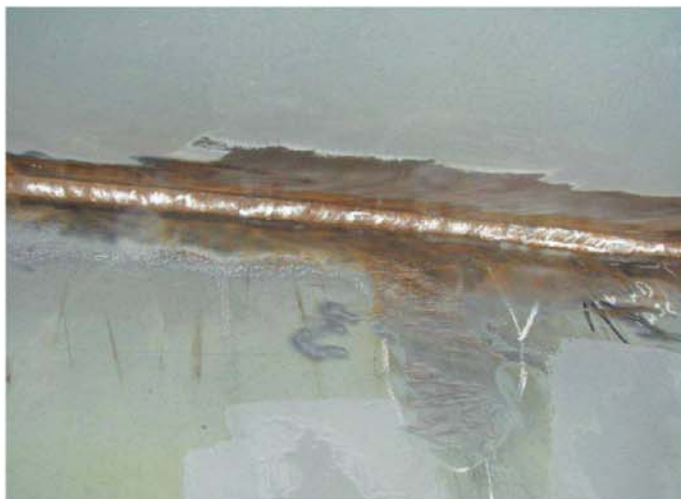
Fig. 4: Butt weld seam grinding
