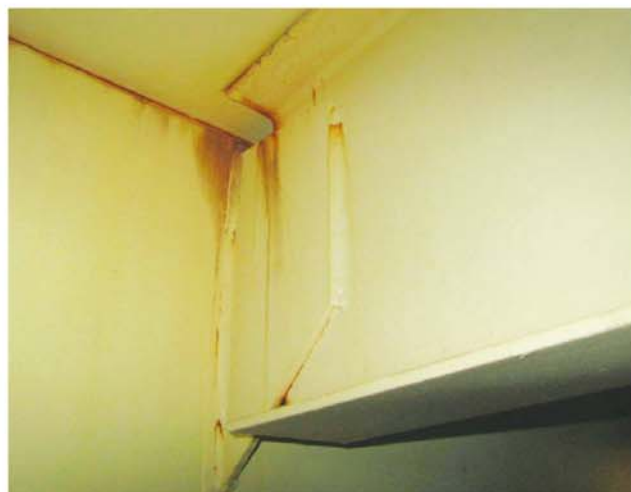
Fig. 5: Non-sealed lap weld at roof support showing problems resulting from open (non-sealed) side
