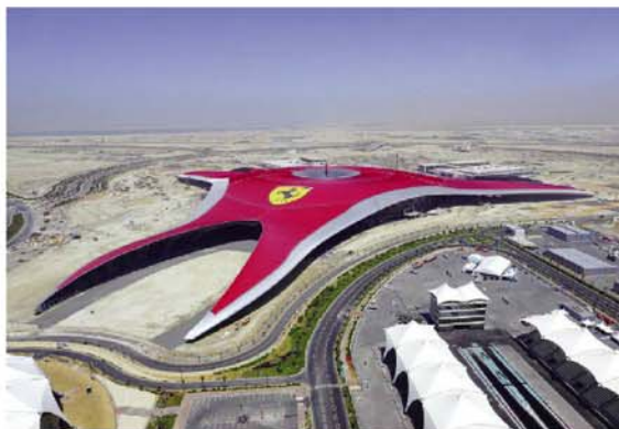
UV resistance from a fluoropolymer coating on the roof of the Ferrari World Theme Park in Abu Dhabi, UAE.
