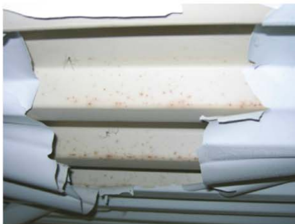
Fig. 1: Extreme delamination of the dry fall coating from the original alkyd on the interior roof panel Photos courtesy of the author.
