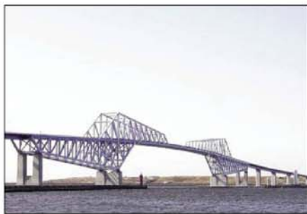
Japan's new Tokyo Gate Bridge is protected with a system that includes a fluoropolymer topcoat.
