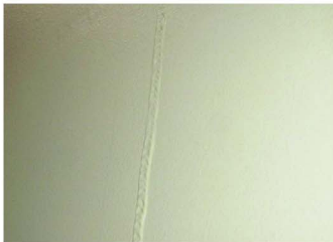
Fig. 8: Coated vertical hand-welded seal seam of butt weld
