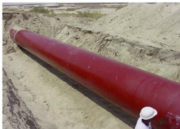
Fig. 3: Buried FBE pipe was found in good condition after 22 years in service in dry sand.
