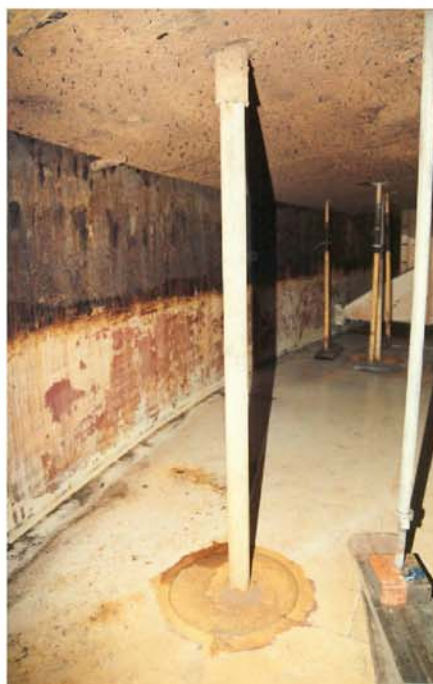
Under floating roof before surface prep
