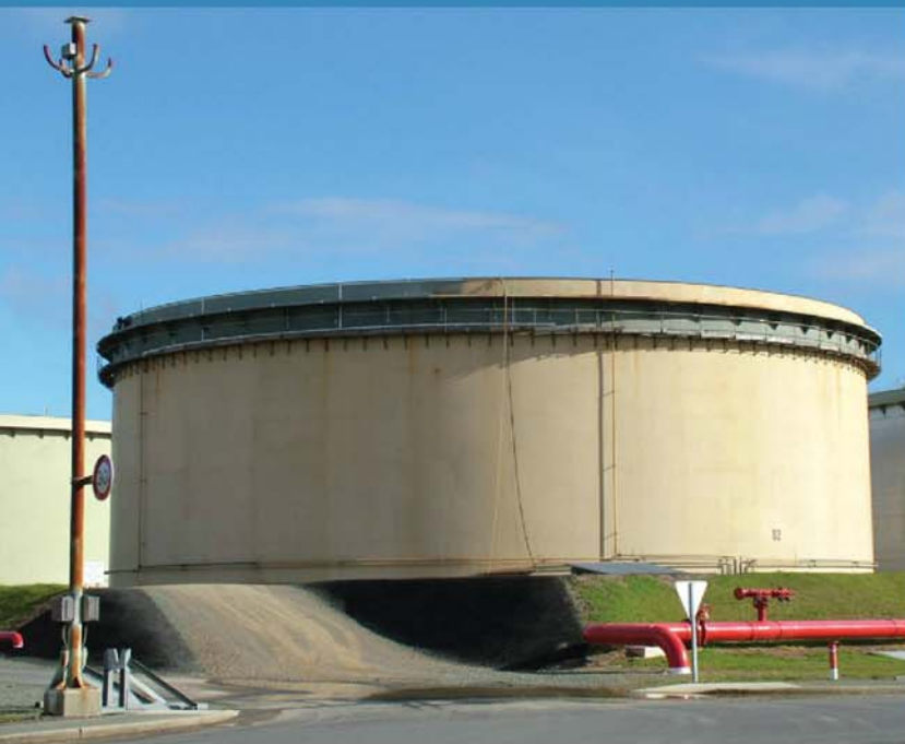
Outside view of Bunker C crude oil storage tank with a floating roof. Surface preparation of the tank interior will be followed by application of a vinyl ester coating. All photos courtesy of Sauereisen
