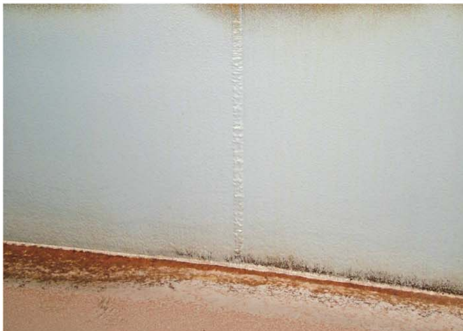
Start of vinyl ester coating on wall above floating roof
