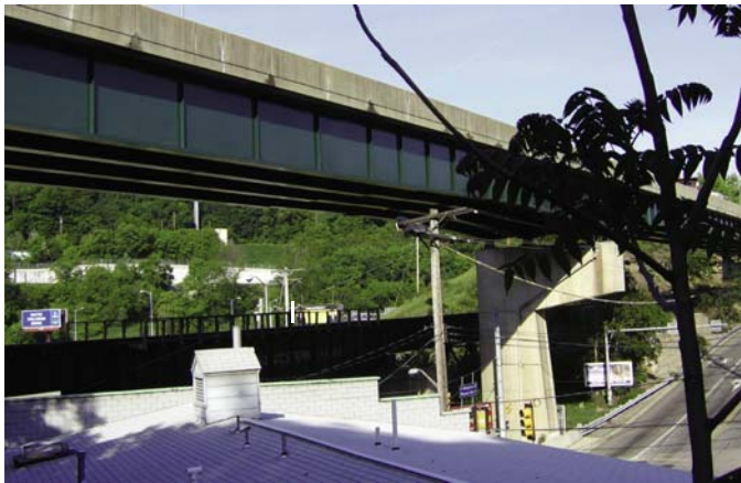
Fig. 4: SSPC-SP 10/organic zinc/epoxy polyamide/acrylic polysiloxane Photos courtesy of International Paint LLC
