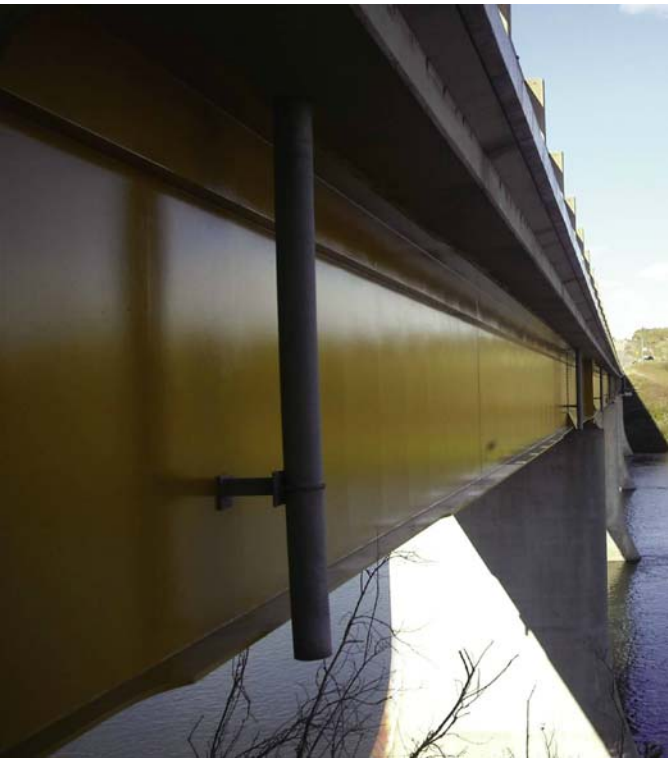
Fig. 6: SSPC-SP 6/organic zinc/polyaspartic urethane
