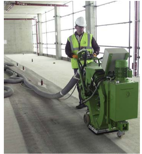
Fig. 6: Shotblasting machine removing surface laitance
