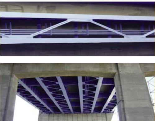
Fig. 5: SSPC-SP 10/inorganic zinc/epoxy/polyurethane on sides, and inorganic zinc/epoxy/polyaspartic polyurethane underneath
