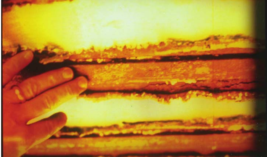
Fig. 7: Condition of the coating on the underside of the viaduct before brush-off blast cleaning
