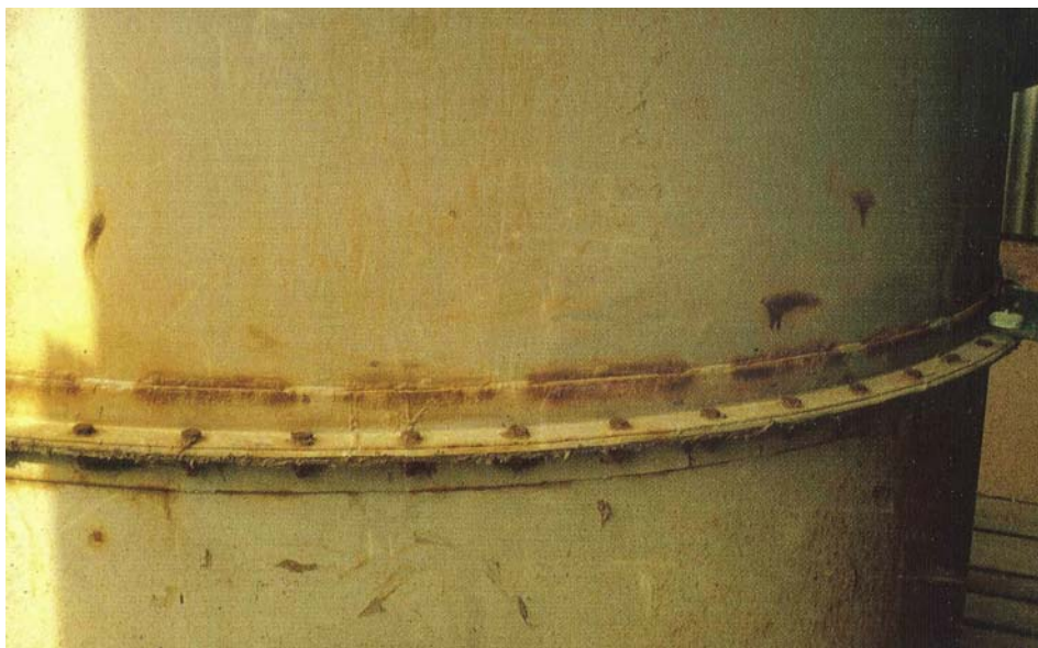
Fig. 3: Severe corrosion is seen at a weld seam. Courtesy of KTA-Tator
