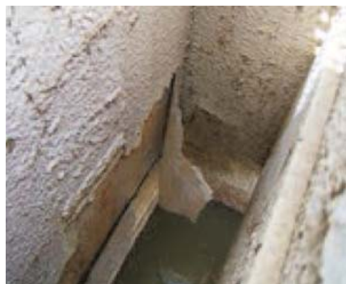
Fig. 2: Delamination failure due to inadequate removal of laitance layer
