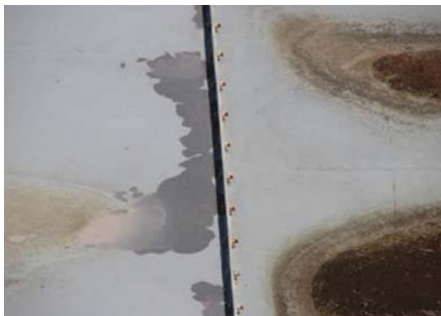
Fig. 1: Exterior surfaces experienced delamination especially on horizontal surfaces. Photos courtesy of KTA-Tator, Inc.
