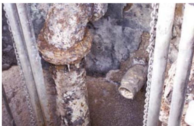
Fig. 1: A wastewater lift station experiencing significant corrosion of concrete, ductile iron, and stainless steel materials. Note the failing coal-tar epoxy that was applied to the concrete and ductile iron materials. Photos courtesy of Tnemec.
