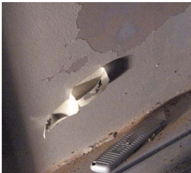
Fig. 2: The adhesion of the coating was variable, even adjacent to large sections of coating delamination
