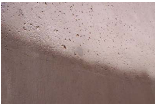
Fig. 4: Properly prepared concrete (above) and concrete repair via a cementitious resurfacing material (below)
