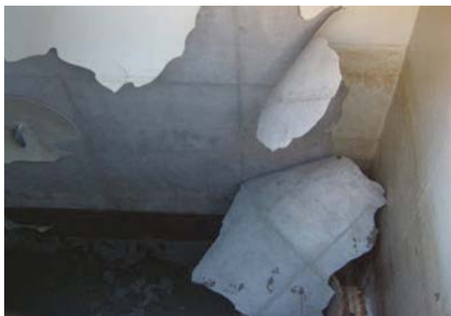
Fig. 3: Delamination failure due to insufficient substrate anchor profile
