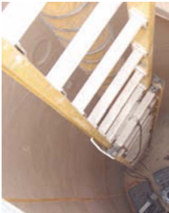
Fig. 5: Finishing touches on a rehabilitated wet well.
