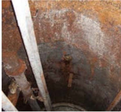
Fig. 4: Corrosion and surface cracking in concrete wet well.
