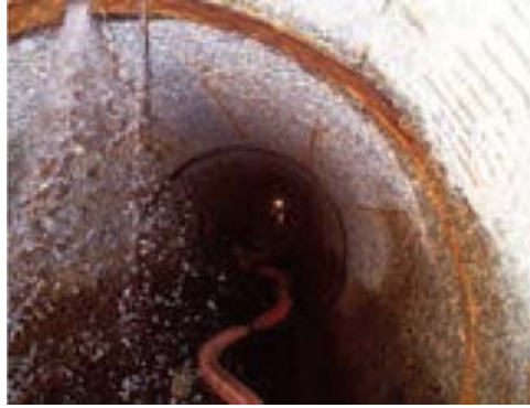
Fig. 2: Active water inflow and infiltration in tunnel.
