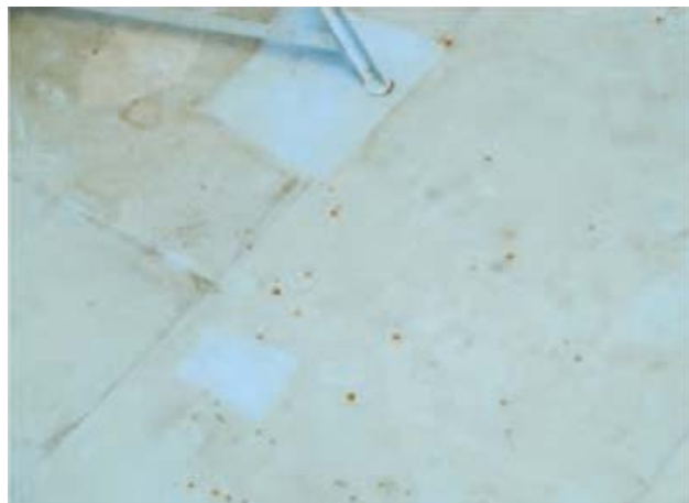
Fig. 3: What appeared to be pinpoint rust on the tank floor was actually embedded metallic fragments in the lining.
