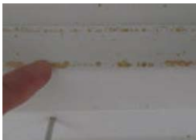
Fig. 6: Typical corrosion/rusting along edge of corrugated roof deck.
