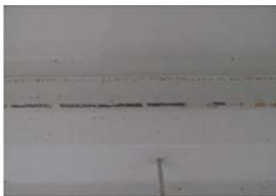
Fig. 1: Typical corrosion/rusting along edge of corrugated roof deck. All figures are courtesy of KTA-Tator.
