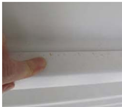
Fig. 3: Area of lesser corrosion on the roof deck.
