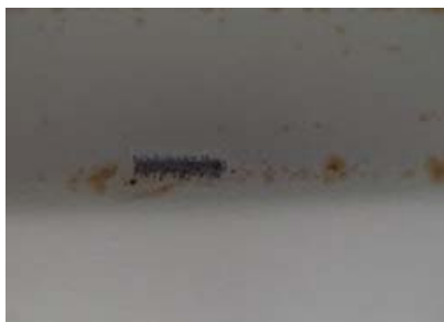
Fig. 2: Rusting on roof deck where coating was removed showing corrosion (black color) in the steel.
