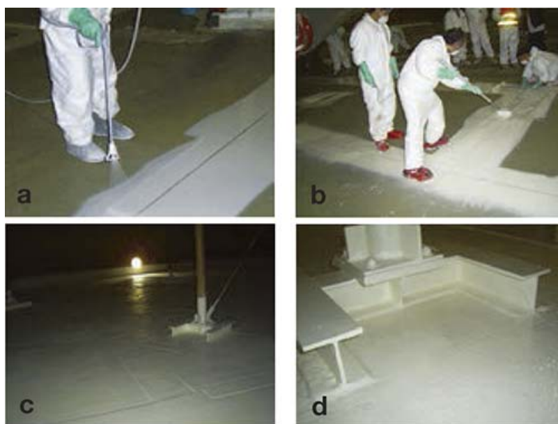
Fig. 3: Lining application: (a) resin application, (b) rolling in fiberglass mat, (c) completed floor and (d) roof stands.
