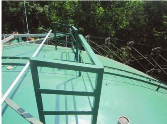
Fig. 11: Antennas reinstalled on tank after coating system cured.
