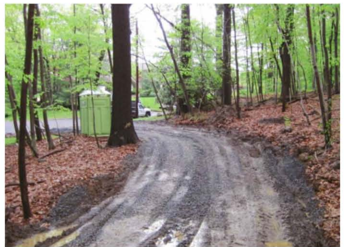
Fig. 3: Crushed stone, fabric were needed to stabilize ground, but it was still difficult to traverse.
