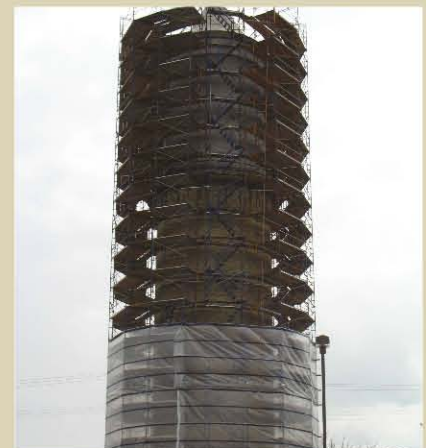
Self-supporting scaffolding and containment.
