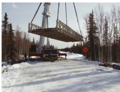
Bridge being lifted from abutments
