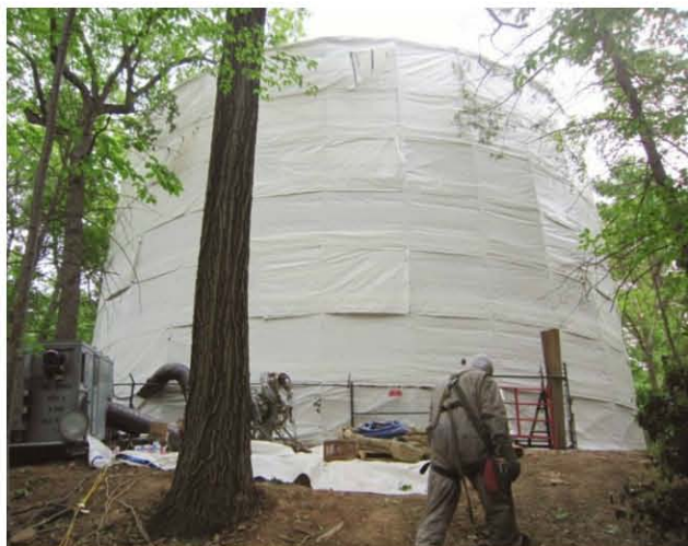
Figs. 9 & 10 (left and right): Longer work days helped crew blast and coat exterior on time.
