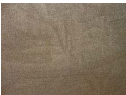
Fig. 8: Blast cleaned floated mortar repair.
