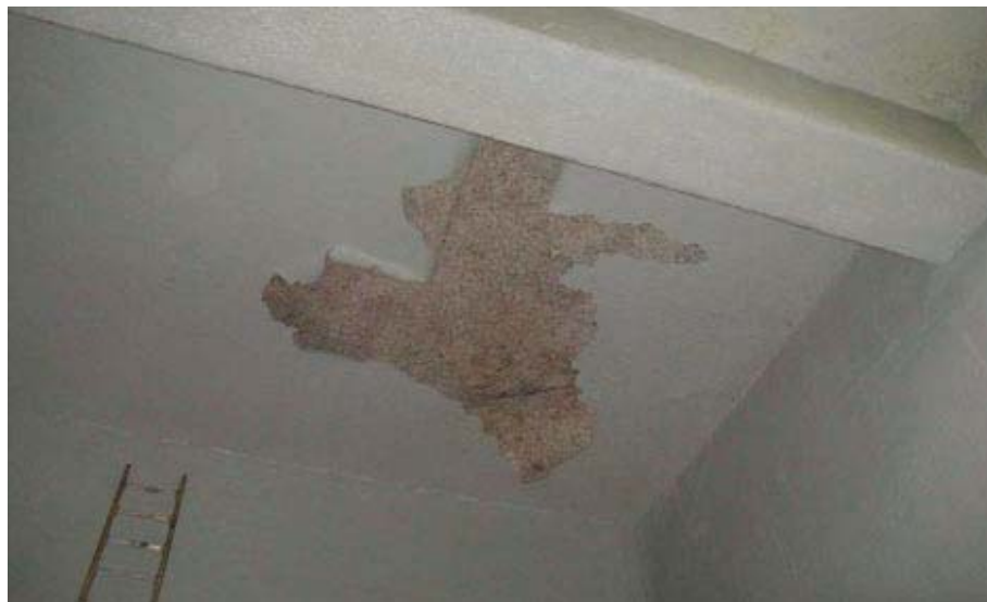
Fig. 3: Large area of lining delamination on ceiling.
