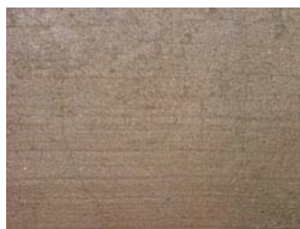
Fig. 9: Blast cleaned repair mortar that was broom finished.
