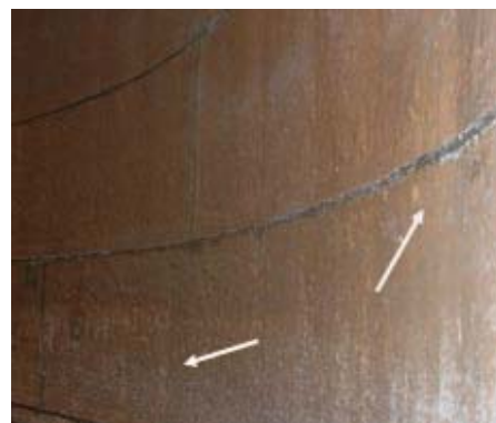
Fig. 12: Blistering and disbondment of lining on lower part of concrete wall of sludge tank with walls built 30% below grade.
