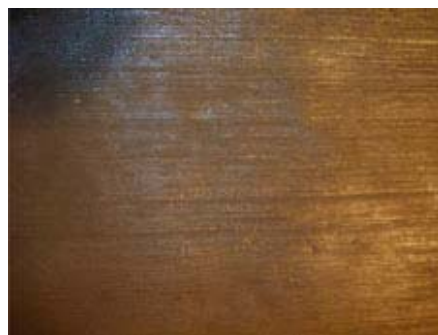
Fig. 7: Typical broom finish on cementitious repair mortar.
