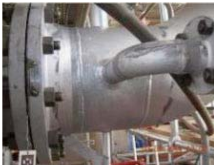
Fig. 30: TMIC applied to protect TSA weld joints
