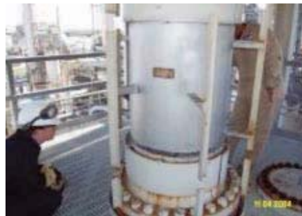
Fig. 31: Inspection of TMIC after 1 year in service showing no coating breakdown or rusting
