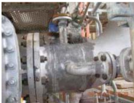
Fig. 29: Preparation of TSA weld joints
