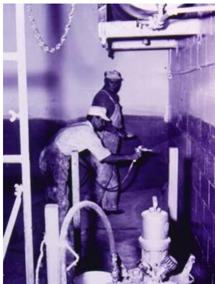
Airless spraying in 1966. While airless technology remains the same today, the industry has seen a lot of other changes since that time, including improvements in worker protection. How far have we come? Photo courtesy of KTA
