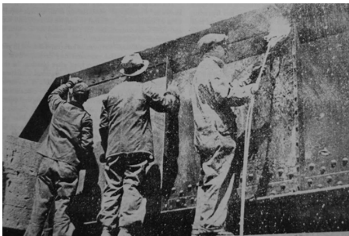
SSPC-SP 4, "Flame Cleaning," was among the surface preparation standards in the 1963 edition of SSPC Volume 2, Systems and Specifications . Flame cleaning (right) was followed by wire brushing (center) and painting (left) while the surface was still warm. Not used in decades, SSPC-SP 4 was withdrawn in 1982. The photo of an old flame cleaning operation appears in the 1996 edition of SSPC Volume 1. Photo courtesy of SSPC
