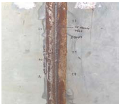
Fig. 3: Coating thickness values along two rusted plate edges. These edges were later cleaned and coated.
