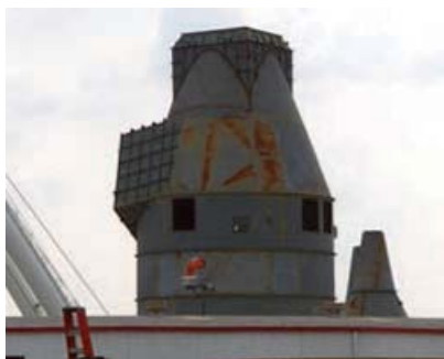
Fig. 2: A second section exhibiting rust staining from the steel crating frames
