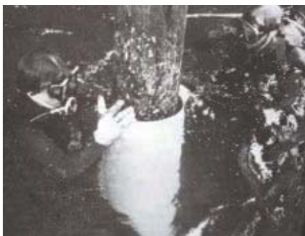
Fig. 6: An early timber pile repair project.
