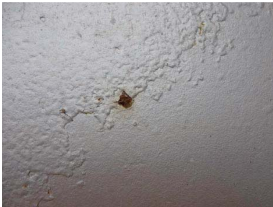
Fig. 3: The rougher coating on the upper left side was thicker, and the old coating system was present. The lower right side had only the new overcoat system. Old coating edges lifted.
