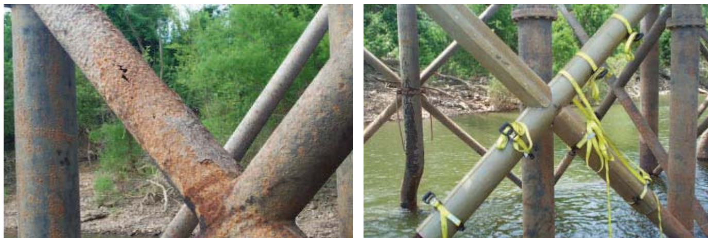
Fig. 7: Inland Steel Water Intake System before and after restoration with fiberglass jackets.
