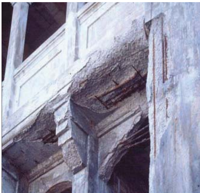
Fig. 2: Reinforcing steel induced concrete spalling likely due to high permeability concrete rapidly carbonating causing corrosion of the imbedded steel.
