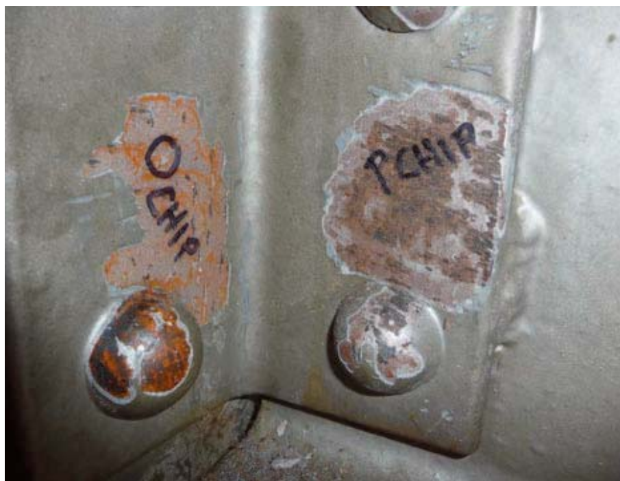
Fig. 2: The left side of the angle shows old primer; the right side does not.
