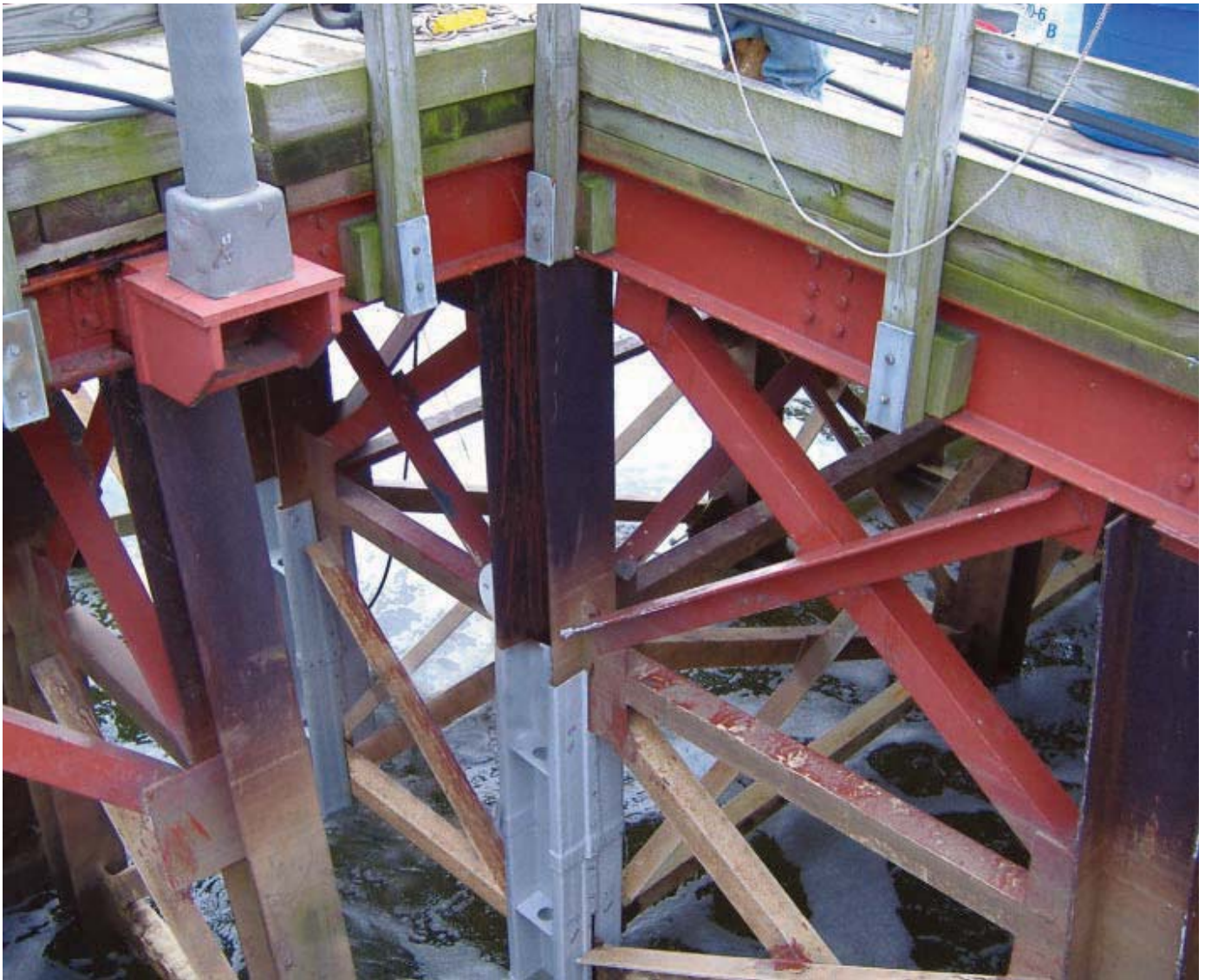
Fig. 1: H-pile repair underway
