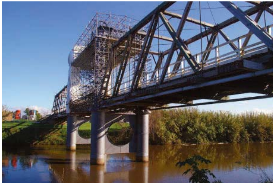
Fig. 6: Shrinkwrap containment of bridge section.
