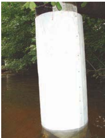
Fig. 9: Steel H pile repaired using a round fiberglass jacket.
