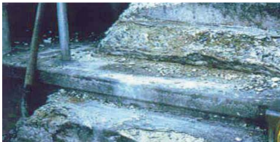
Fig. 3: Deterioration of concrete steps from environmental attack such as acid exposure and deicer scaling. Figs. 2, 3, and 4 courtesy of BASF
