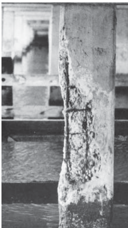
Fig 3.: The first image shows a severely deteriorated pile at the 26th Street Bridge in Norfolk, VA; the second shows the completed restoration, 106 piles in total.
