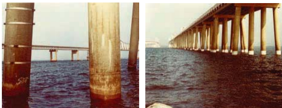
Fig. 4: (left) Piles under the Chesapeake Bay Bridge showed extensive scouring due to conditions; (right): the bridge after the restoration has been completed.
