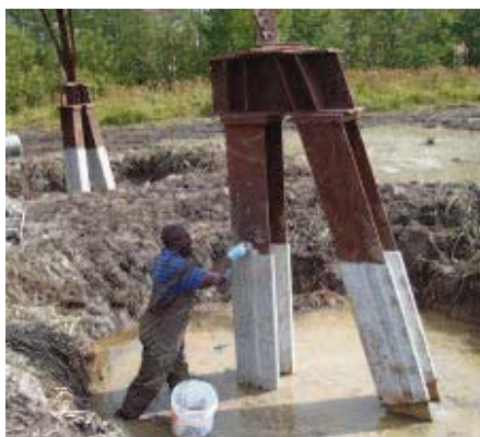
Fig. 8: Steel H piles repaired with an H-shaped fiberglass jacket.
