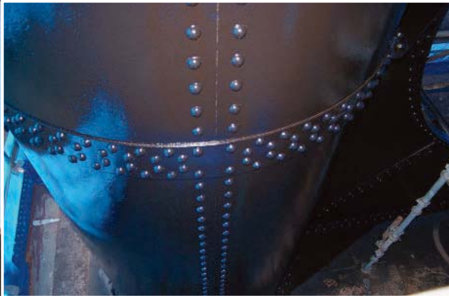
Fig. 7: Riveted and coated cast iron pier.
