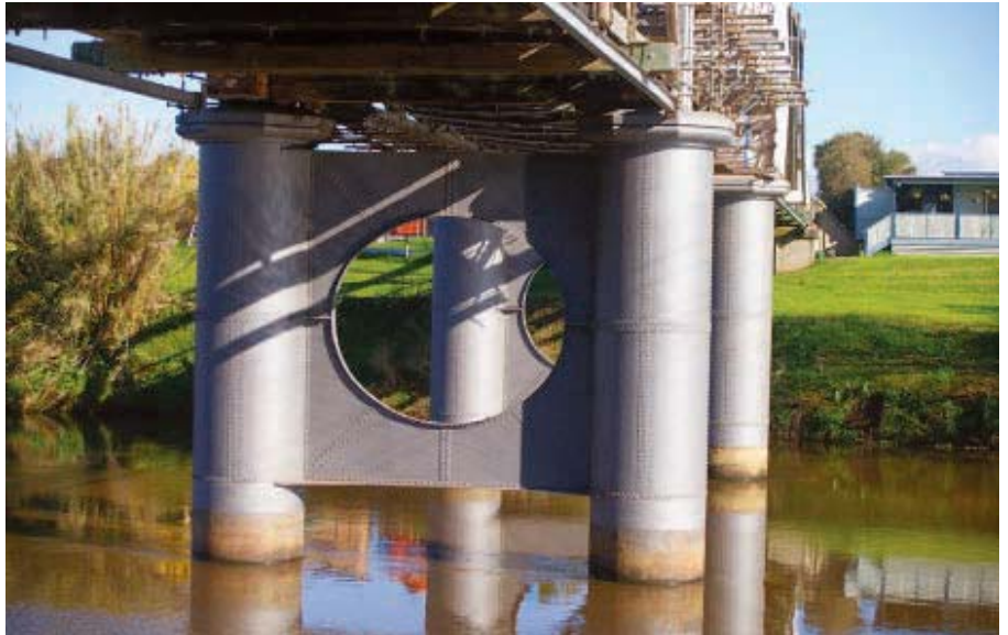
Fig. 3: Finished twin cast iron cylinder piers.
