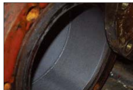
Fig. 4: Pipe wall internals after removal of wax, deposits, and mill scale.
