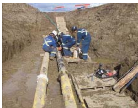
Fig. 8: EnerClear personnel inspecting the final application of coating for DFT adhesion and cure at mid-point spool.
