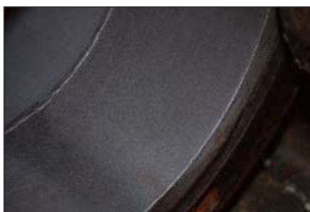
Fig. 5: Final inspection of pipe wall internals prior to running drying agents in preparation for first coat.
