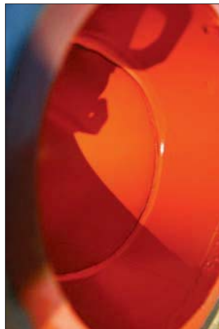
Fig. 7: First coat averaged 3 mils DFT, an additional 2 coats were applied to achieve the required 10-12 mils DFT.
