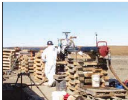
Fig. 6: Worker monitoring back pressure on receiving end as coating run is in progress.
