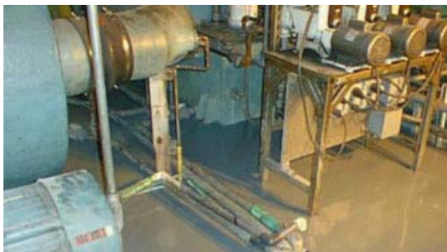
The sump seen here is lined with novolac epoxy polymer concrete.
