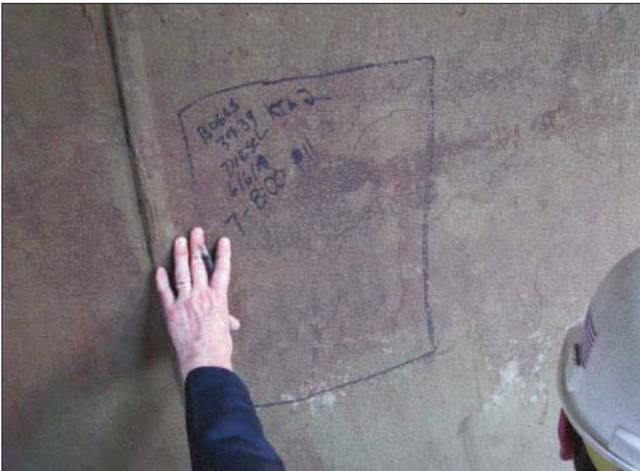
Fig. 5: Sample marked for cutout. All samples were marked in this fashion. This sample was taken from a fiberglass-lined steel tank. Adhesion was excellent.
