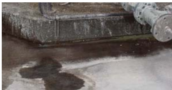
Pump pad, floor, and dike wall, all of polymer concrete, are exposed to concentrated sulfuric acid spillage and leaks on a continuous basis.
