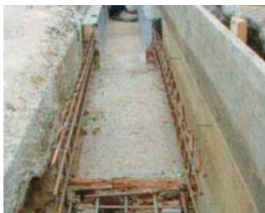
Polymer concrete cast in place to form trenches to carry concentrated sulfuric acid to neutralization tank.
