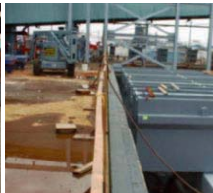
Cells, support beams, floor pad and containment wall all cast from Bis A polymer concrete.
