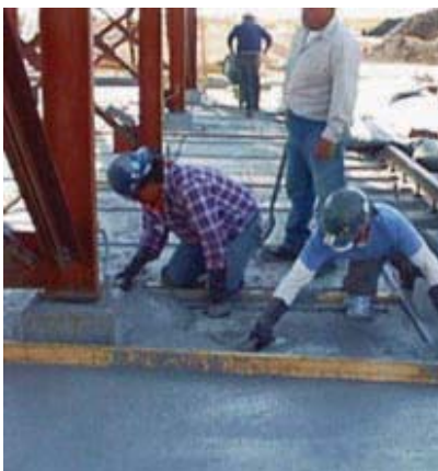
Potassium silicate PC being installed under and around railcar unloading pad.
