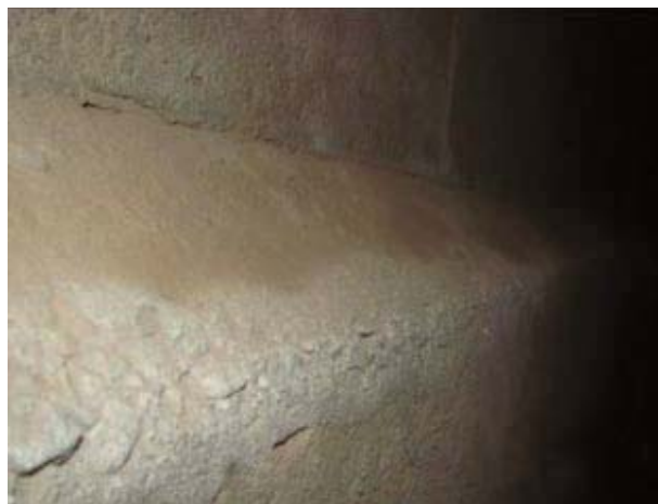
Fig. 1: Substrate after sandblasting and before sealer coat application
