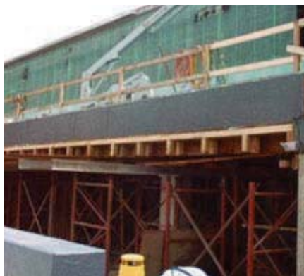
Formed polymer concrete wall and part of cell.
