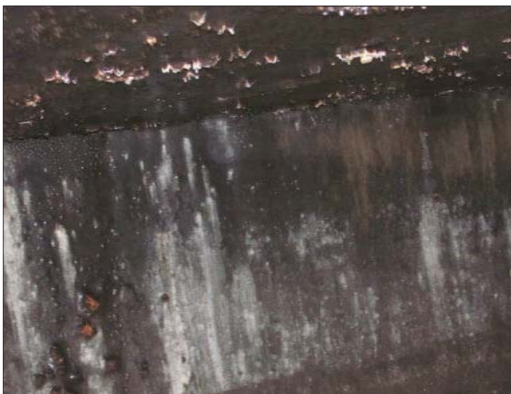
Fig. 6: The roughing filter wetwell had both large and small blisters ( \frac{1}{16} inch to 2 inches in diameter) on the walls and roof. Some had opened up to expose soft concrete.
