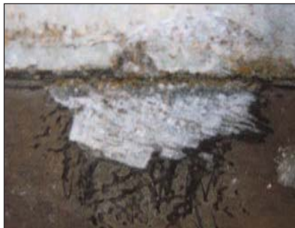
Fig. 2: Above the water line, the coating was tightly bonded and had to be chipped off with a chisel.
