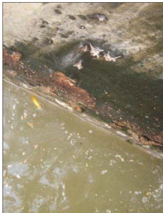
Fig. 1: Condition of the coating at the primary effluent wetwell hatch. Coating failures were observed only at the water line area. Photos courtesy of KTA-Tator
