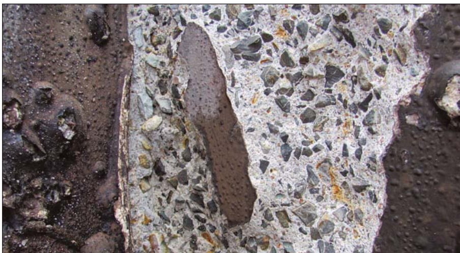
Fig. 3: Typical condition of the coating below the water line after pressure water washing. Note the blisters that cover the surface of the coating. Also note the exposed aggregate after the degraded coating and concrete were removed.
