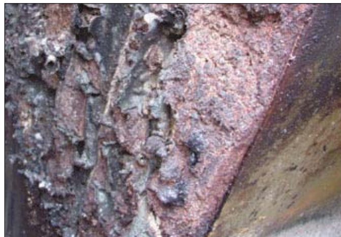
Fig. 5: An example of the condition of the wetwell walls where the coating had lifted and had broken apart. The underlying concrete is extremely soft. The coating is brittle.
