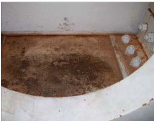
Figs 1 and 2: Rusting on bolted connection in girder ends. Note moisture and/or ponding water. Photos courtesy of KTA-Tator, Inc.
