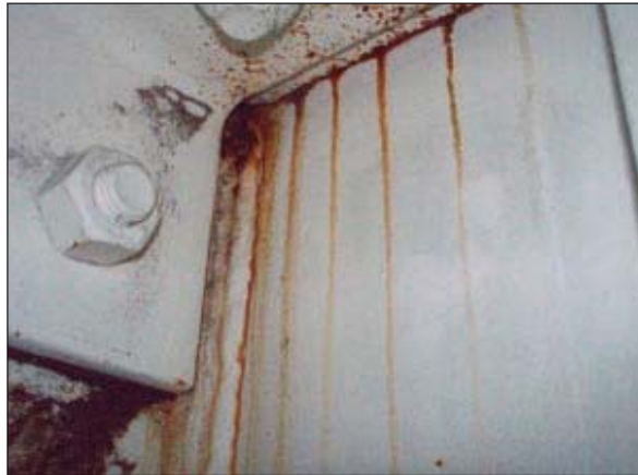
Fig. 5: Indications of moisture leaking from the top crevice of box girder.
