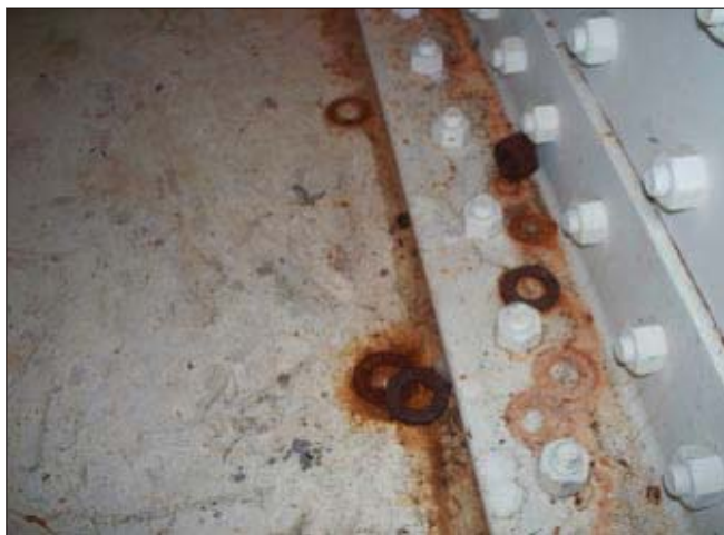
Fig. 6: Metal washers, metallic shavings, and nuts rusting and staining the coating.
