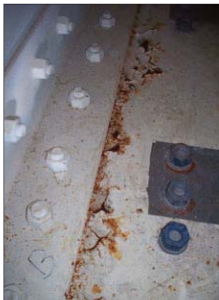
Fig. 7: Blistered and peeling coating on girder floor. Note that blisters are more concentrated along the crevice of the bolted angle to the floor.
