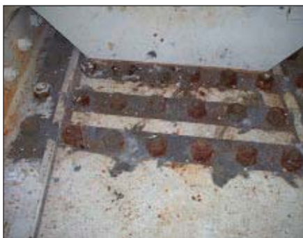
Fig. 4: Uncoated bolts rusting
