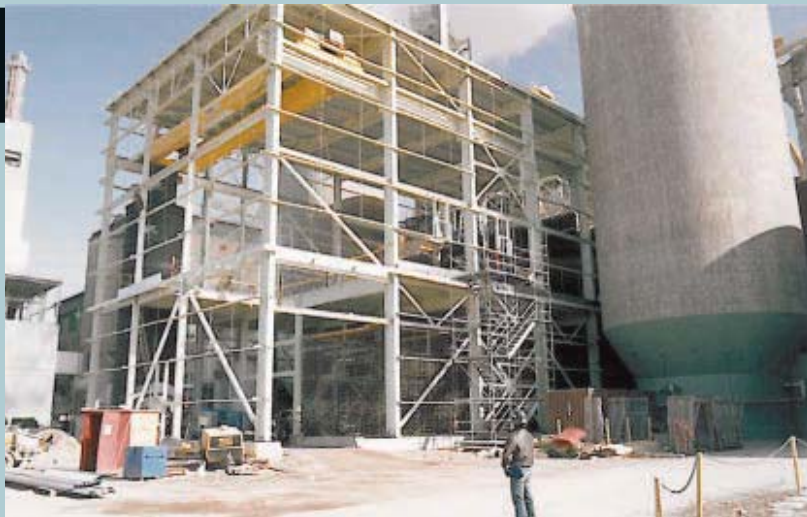
Erection of structural steel. Photos courtesy of Tembec Industries
