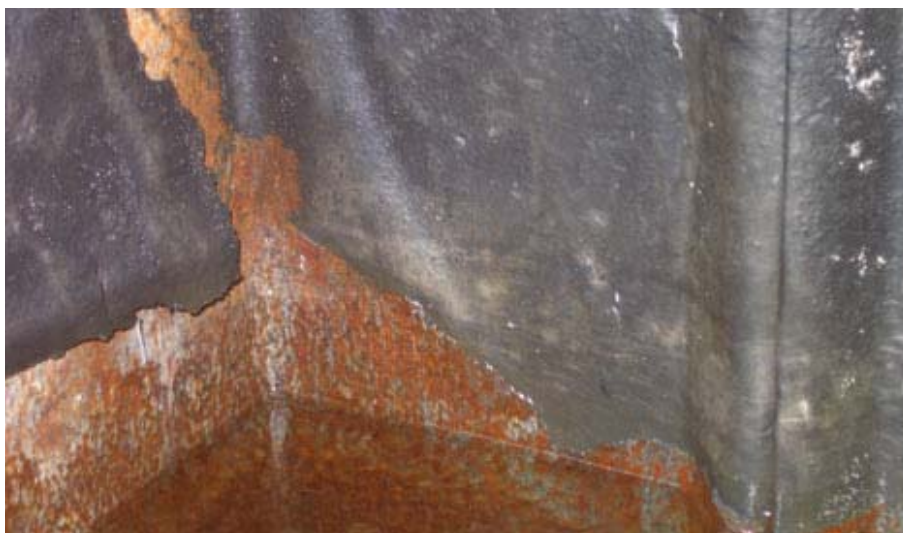
Large areas of delaminated coating in the splash zone. Photos courtesy of the author
