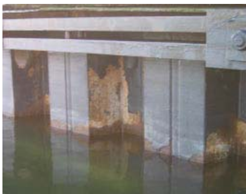
Delaminated areas on new coating viewed at low tide.
