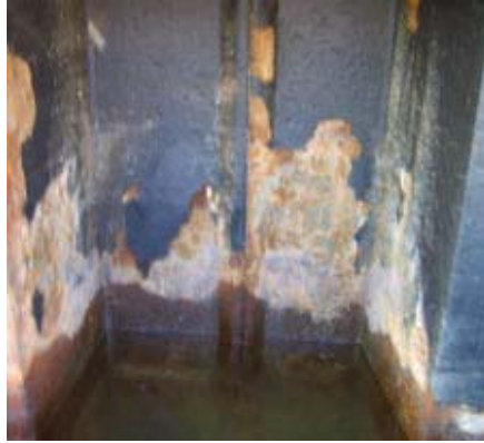
Close-up of delaminated areas on new coating. Whitish areas are alkaline deposits from cathodic protection.
