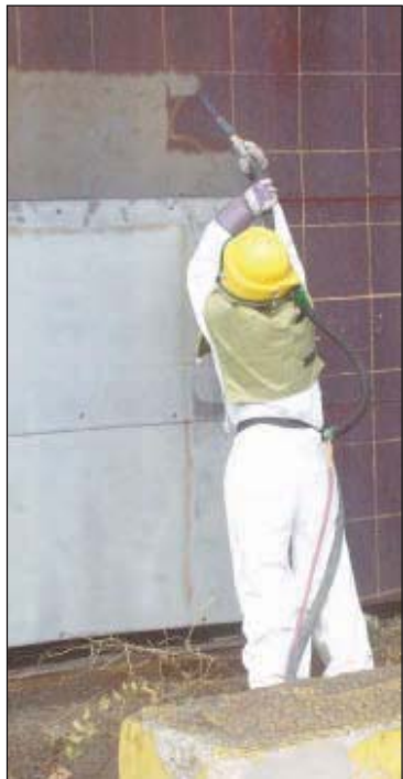
Productivity test, conducted under third-party guidance, on heavily pitted and rusted steel structure at a steel mill. Round and angular abrasives were tested for productivity and usage.
