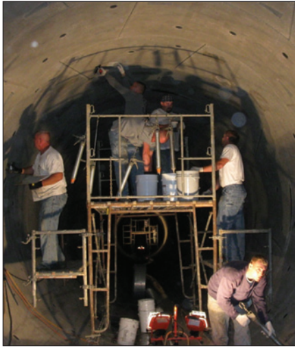
Fig. 10: Filling chamfer area of segment joints and covering grout port caps.
