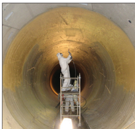
Fig. 3: Application of fiber-reinforced 100% solids epoxy coating
