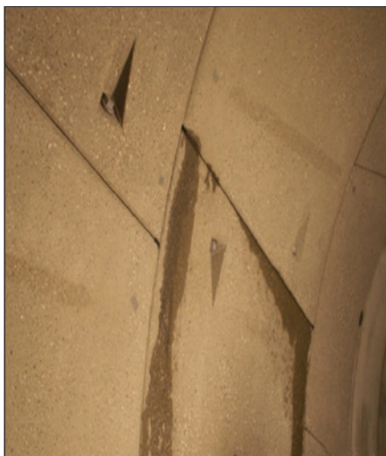
Figs. 6 and 7: Bolted ring sections after installation in the tunnel. The dark discoloration on the left was typical of a leaking segment joint (left); bolt pocket ready to be filled (right).
