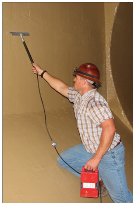
Fig. 12: Holiday detection being performed on the completed coating system
