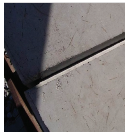
Fig. 5: Close-up of unfilled segment seam.
