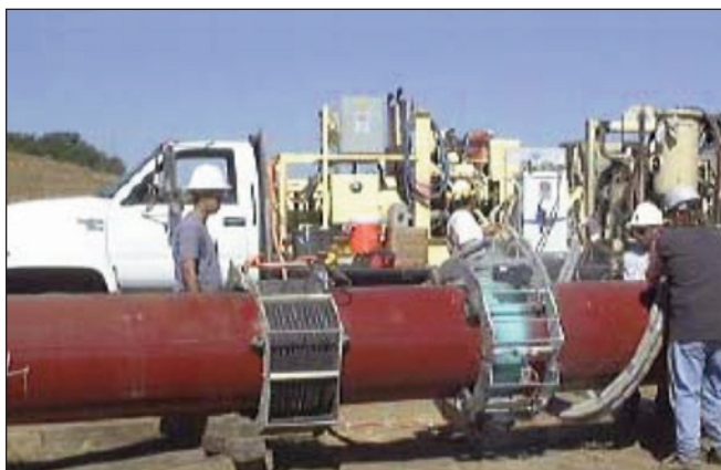
Fig. 5: Heating of a pipe string girth weld area.
