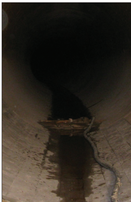
Fig. 13: After remedial repairs, stainless steel plating was installed to protect against erosion from scouring (Table 5, p. 48).
