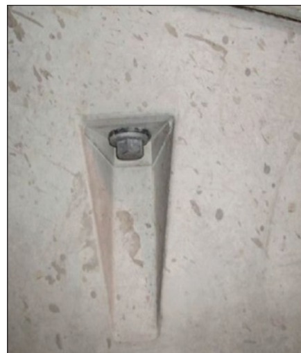
Figs. 6 and 7: Bolted ring sections after installation in the tunnel. The dark discoloration on the left was typical of a leaking segment joint (left); bolt pocket ready to be filled (right).
