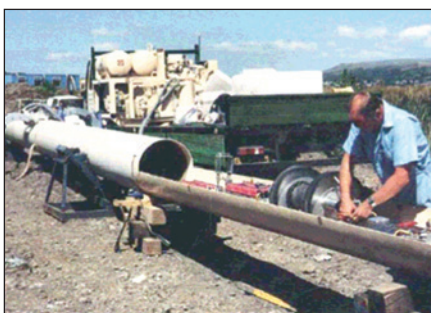
Fig. 2: A typical pipe string being prepared for the launching of a robotic crawler.
