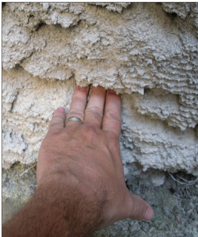
Fig.2: Existing shotcrete surface ready to be resurfaced and protected with fiber-reinforced lining. One of four conditions (Table 3, p. 46).
