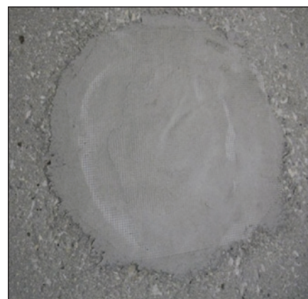
Figs. 8 and 9: Photos show one of over 4,000 grout ports to be addressed before applying a protective lining. The discoloration around the port on the left indicates water infiltration before being covered. The grout port on the right has been covered and embedded with fiberglass, waiting for resurfacing topcoat.
