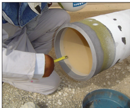
Fig. 1: Cutback portion that was abrasive blast cleaned. The lighter portion of the coating shows what was "feathered" (roughened).
