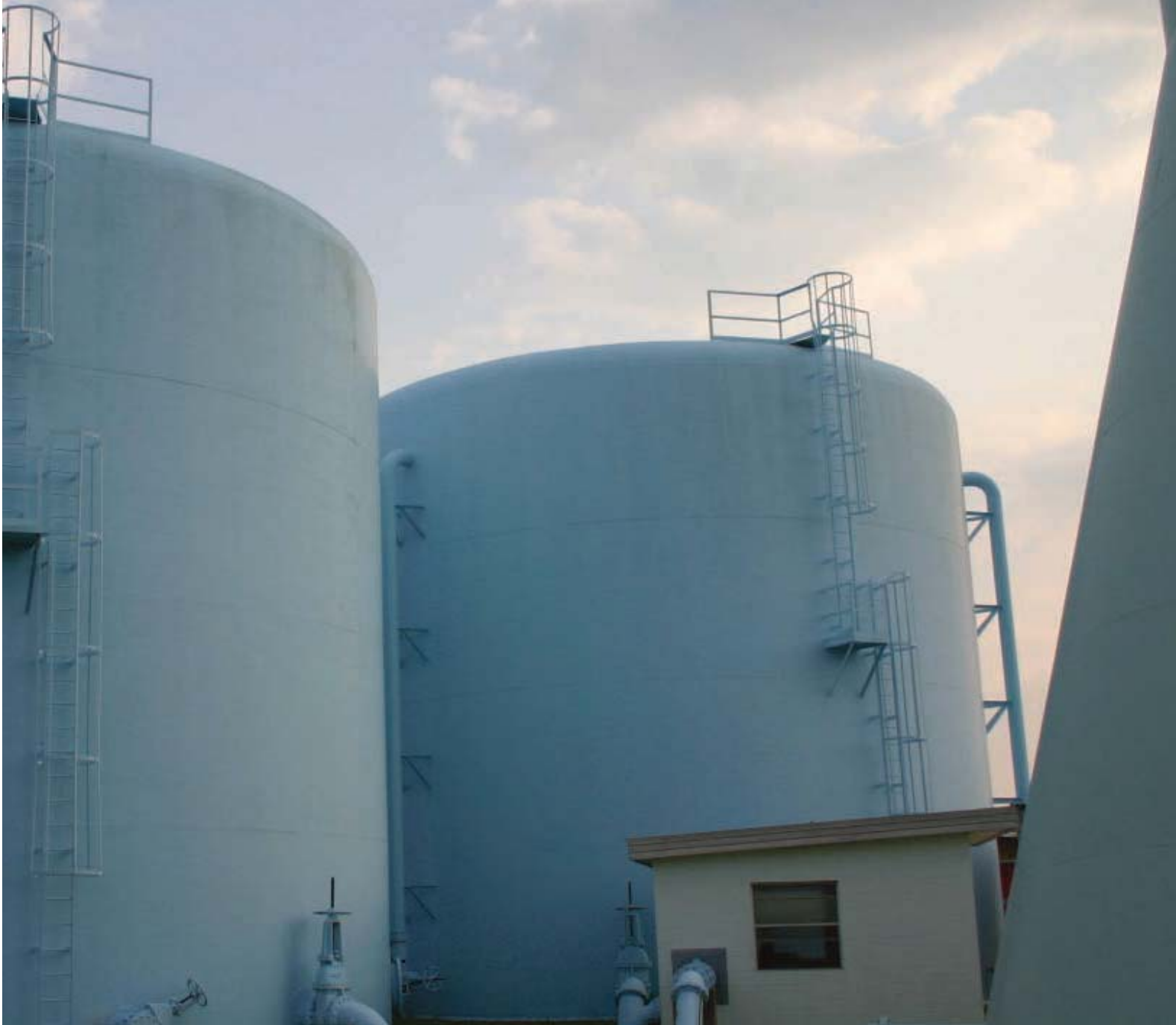
Surface preparation requirements for the interiors of most water storage tanks (e.g., above) are typically stringent; requirements for preparing demineralized water tank interiors can be even more demanding.
