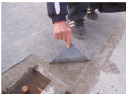
Fig. 3: Polyurea delamination on jobsite in hot summer and cold winter
