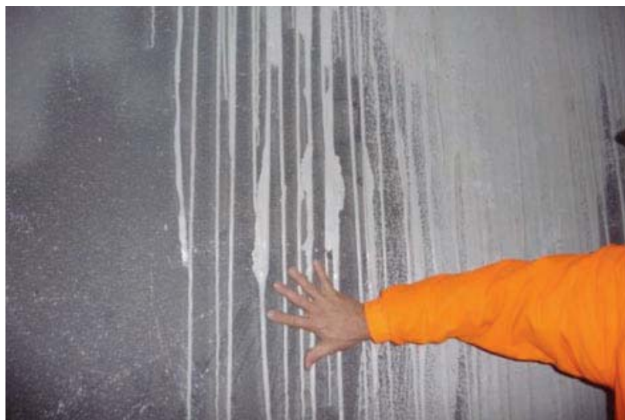
Fig. 2: An example of the size and degree of coating runs present on portions of the bottom shell wall.
