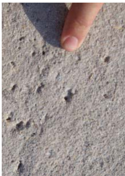
Fig. 2: Concrete surface defects after shot blasting
