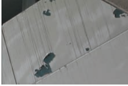
Fig. 3: Compromised coating adhesion on solid wall panels
