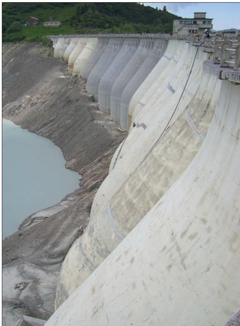
Gray and orange horizontal stripes are crack repair areas on Girotte Dam in France Photos courtesy of WIWA Wilhelm-Wagner GmbH & Co. KG ©2010
