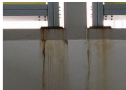
Fig. 10: Extensive rust bleeding on steel footings supporting wall panels
