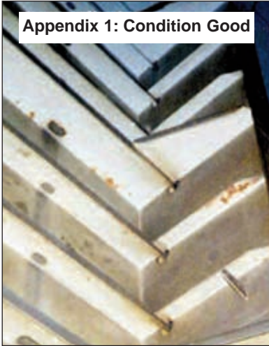
1% SCATTERED CORROSION
