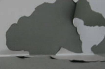
Fig. 2: Split in primer on solid wall panels
