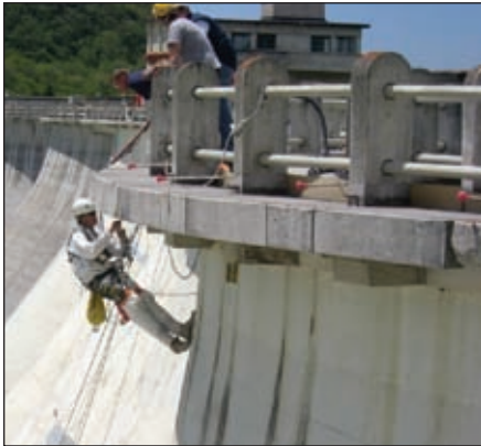
Worker had to rappel to repair cracks
