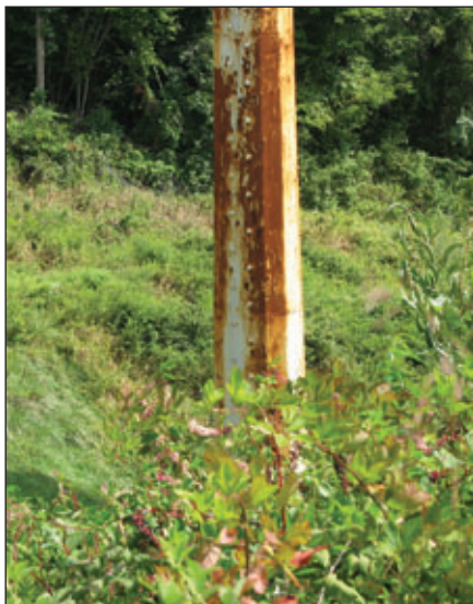
Fig. 3: On some older steel structures, the steel footing is in direct contact with the ground.
