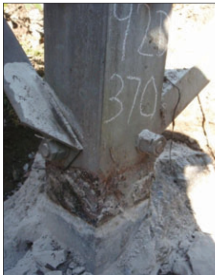
Fig. 2: The below grade surface, often called the footing or foundation, is a major area of maintenance concern. Figs. 1-5 courtesy of the author.
