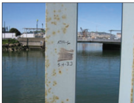
Fig. 3: The substrate had been profiled, but only two coats of paint were visible with the naked eye. The gray primer appeared to be missing.
