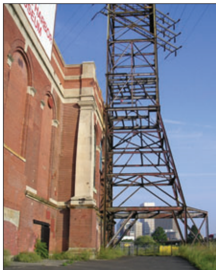
Fig. 4: Steel latticework can trap moisture, causing accelerated corrosion.
