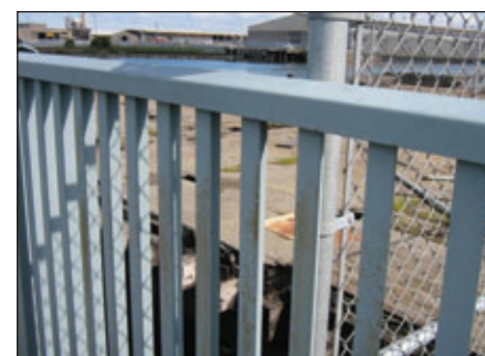
Fig. 2: An example of the condition of the handrail on the east side of the bridge and along the southern end of the west side. At this location, rust was observed on almost every picket.
