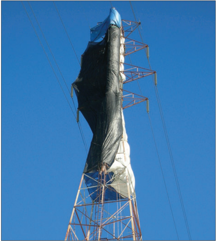
Fig. 6: State and Federal laws require containment of lead paint to protect workers, residential areas, and the environment. Courtesy of Savannah River Crossing, Georgia Power Company
