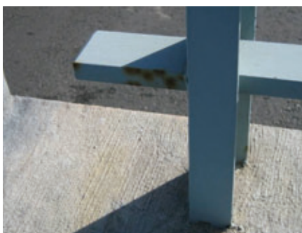
Fig. 5: Typical condition of the end pieces on the guardrail showing general rusting.
