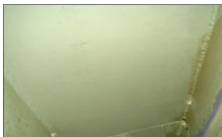
Fig. 7: Excellent condition of the coating after inspection, with the original gloss still present.
