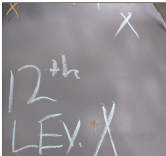
Each level of the scaffold was marked.
