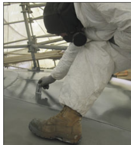
Wet film thickness as well as dry film thickness was measured throughout the work.
