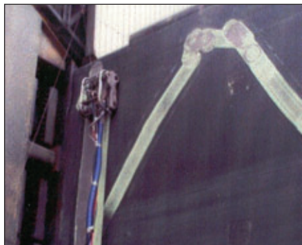
Fig. 6: UHP water jetting crawler on gate during repair work.
