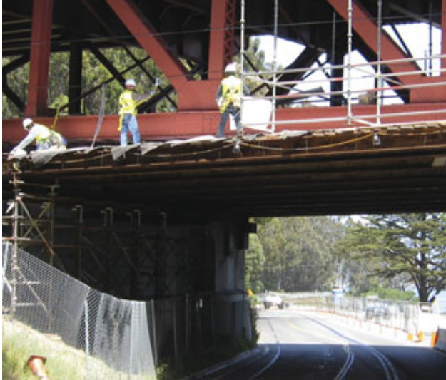
Fig. 4: Workers attached to a job-installed cable during scaffold erection. Training for scaffold users differs from that for scaffold erectors. Courtesy of the author
