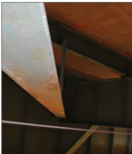
Fig. 3: Corrosion on bottom flange
