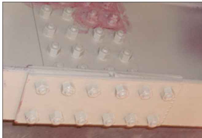
Fig. 9: Bleeding and color migration of the primer through the topcoat during striping of the topcoat.
