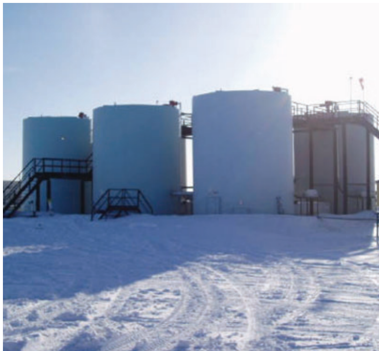
Fig. 4: Un-insulated tanks in Canadian oil patch—hot cargo with a large cold wall effect in winter. Lined with Coating A (a two-coat epoxy novolac) at 12-18 mils total DFT. No coating breakdown in real life performance after 15 years.
