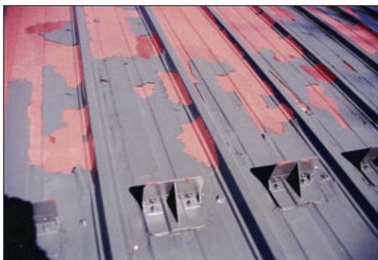
Fig. 2: Close-up of delaminating topcoat
