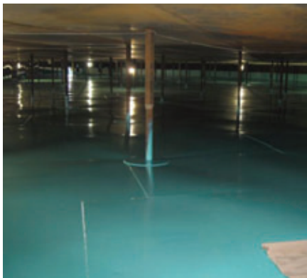
Interior tank painting, Hardisty, AB, Canada Courtesy of Park Derochie Coatings Ltd.
