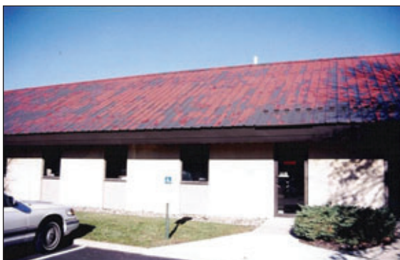
Fig. 1: Overall view of coating roof failure. Photos courtesy of the author
