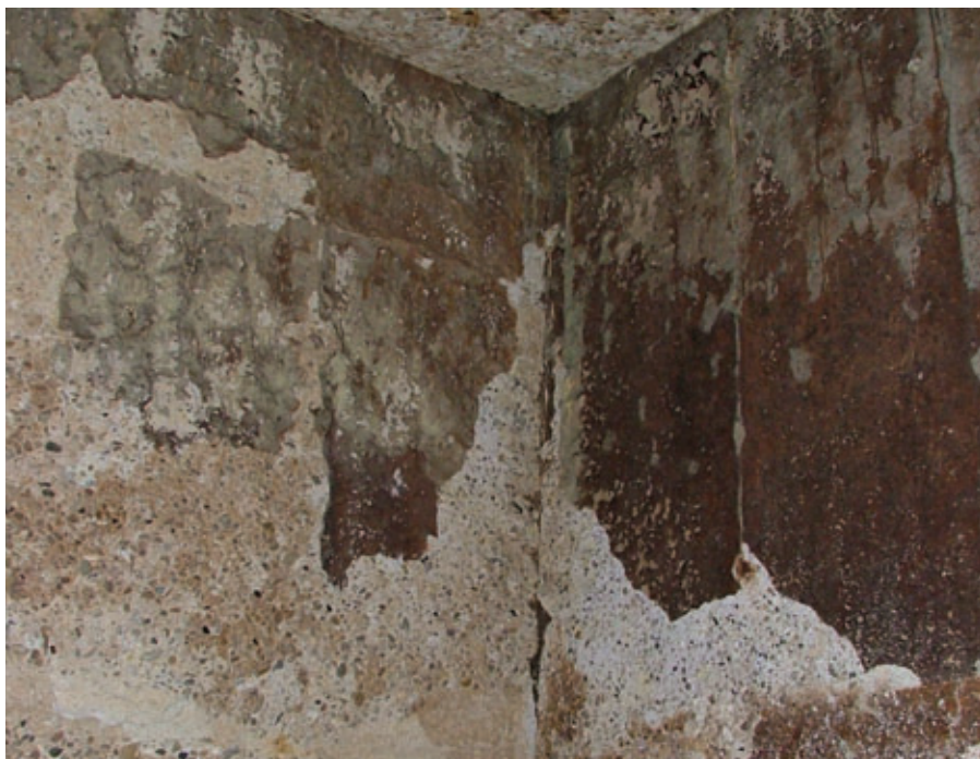
Fig. 4: Grit tank headspace with non-operable odor control system
