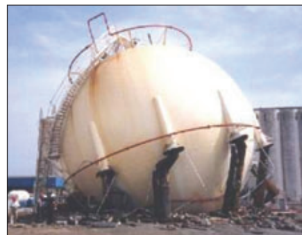
Fig. 11: A sphere collapsed due to undetected corrosion under cementitious PFP. Photo courtesy of International Paint
