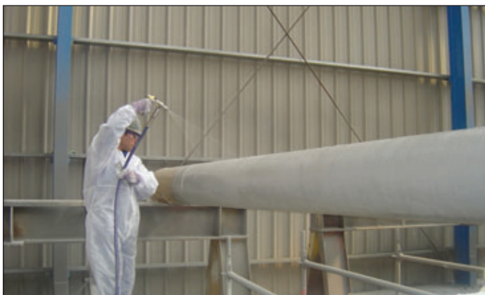
Figs. 5 and 6: Intumescent applied to an offshore platform under construction. Photos courtesy of Disnamair S.A.; WIWA GmbH; and Dragados Off Shore S.A.
