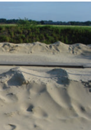
Fig. 4 (Left): Eroded sand berm
