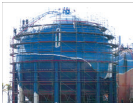
Fig. 9: Coating application on a gas sphere in Tenerife, Spain. Photo courtesy of Disnamair S.A. and Compañía Española de Petróleos S.A.
