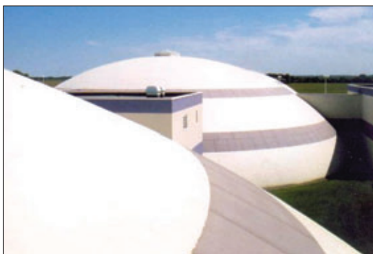
Fig 1: Monolithic Airform Dome Construction was used for this school in the Midwest U.S. Photos courtesy of Thomas Neal
