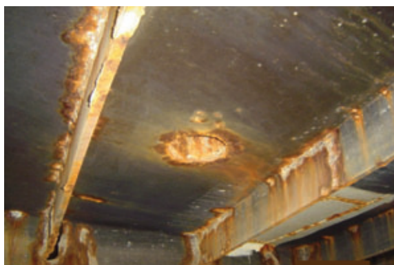
Fig. 5: Extensive corrosion
