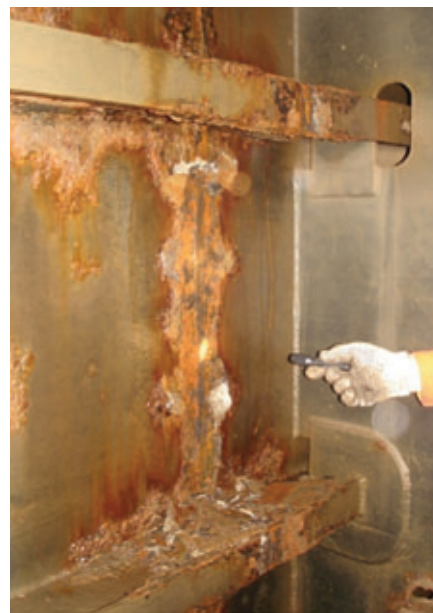
Fig. 7: Corrosion at weld seams
