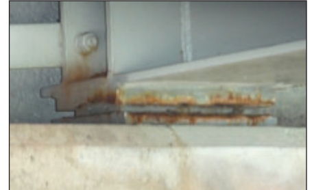
Corrosion at bearing Photos courtesy of the author
