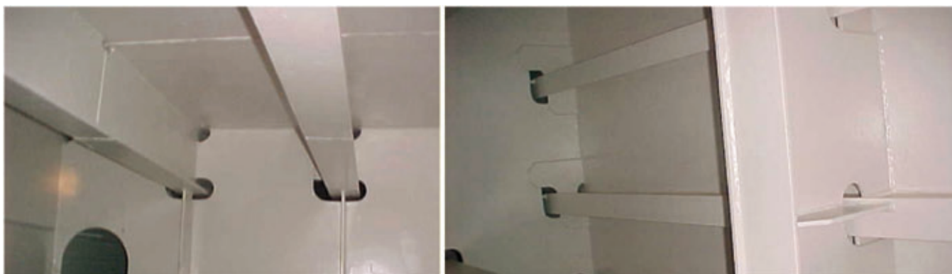
Fig. 10: Final result using hydro-blasting and wet surface tolerant epoxy
