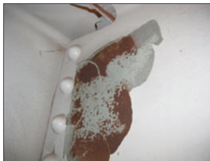
Cracked thick coating overrust
