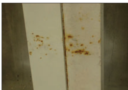
Corrosion at rigging point
