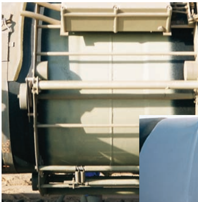
Fig. 5: FJC with epoxy-modified PV applied on 3LPE-coated pipes
