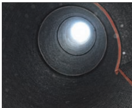
Fig. 3: A view of the stack with lining work complete
