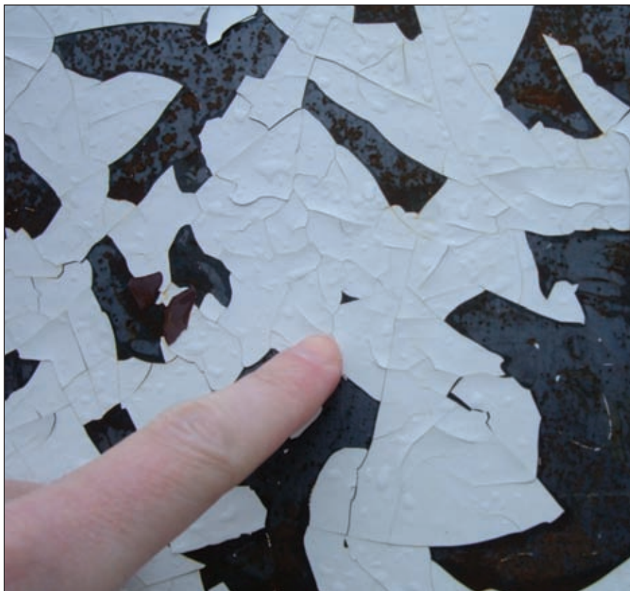
Fig 1: Nearly all of the coating had delaminated or was cracked and loosely adhered to the steel surface. Photos courtesy of KTA-Tator, Inc.
