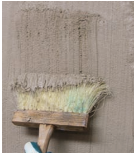
Fig. 1: Typical broom-finished surface
