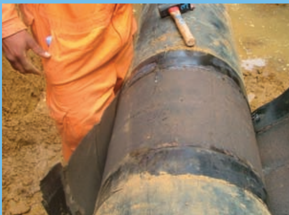
Fig. 1: Lack of adherence of HSS on PE (top) and steel (below) on 18-inch Gabon. All photos courtesy of the authors.
