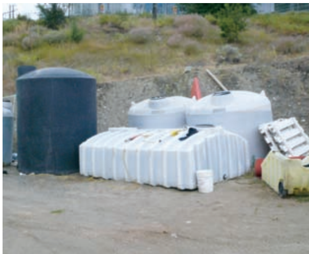
Fig. 6: Holding tanks for used water and paint chips
