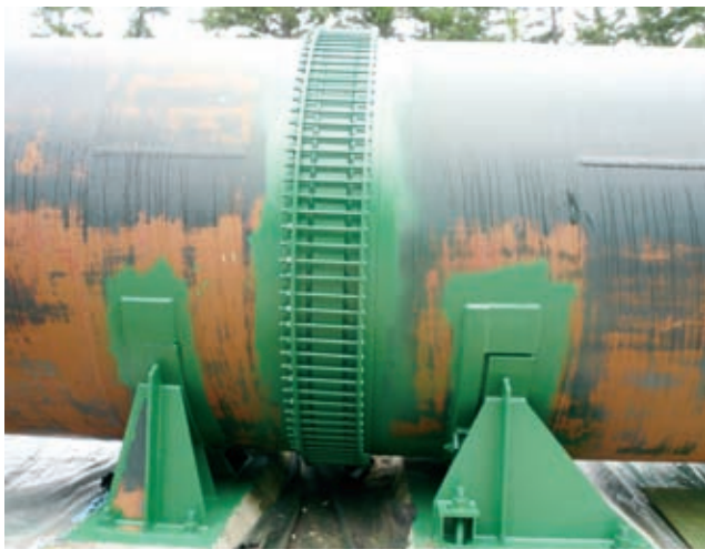
Fig. 11: Full coat of HRCSA adjacent to Dresser coupling
