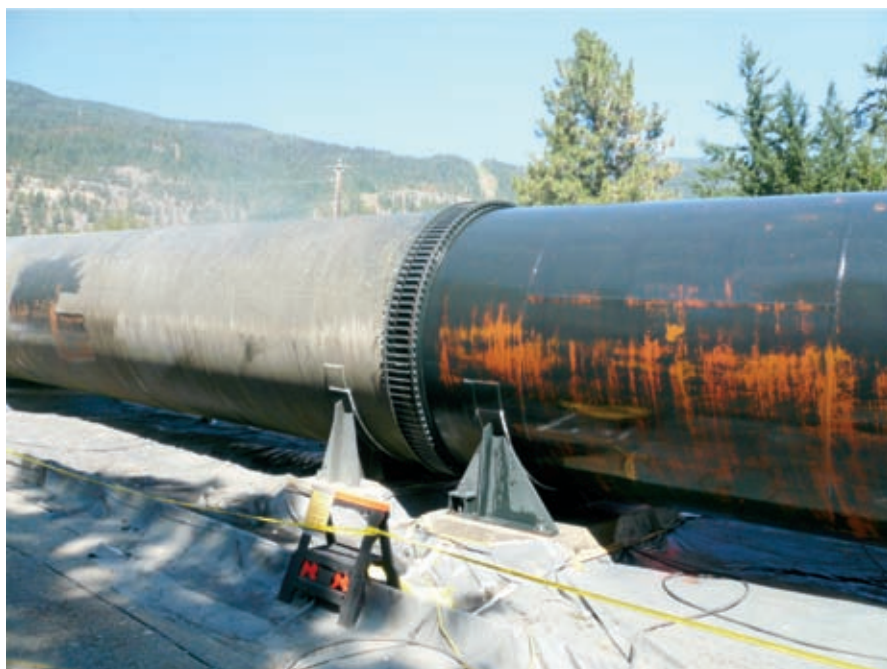
Fig. 5: View of pressure-washed surface and containment system beneath the penstock
