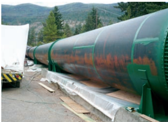
Fig. 14: Containment enclosure to keep drums of HRCSA cool
