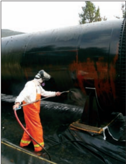
Fig. 4: Surface preparation—pressure washing at 5,000 psi
