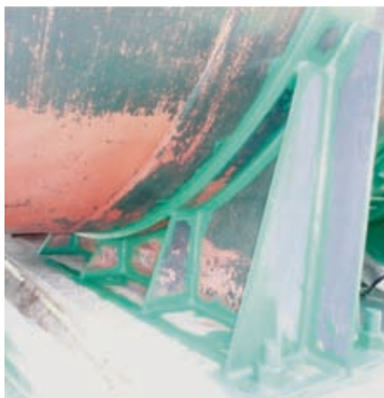
Fig. 10: Stripe coating with finish coat of HRCSA
