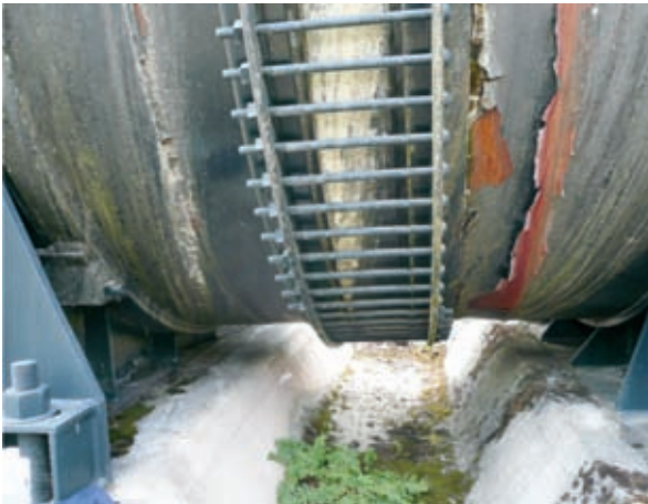
Fig. 3: Deterioration of the original lead-based alkyd paint system
