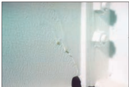
Fig. 5: Excessively thick coating films were commonly found, as exemplified by the "curtain" in this photograph.
