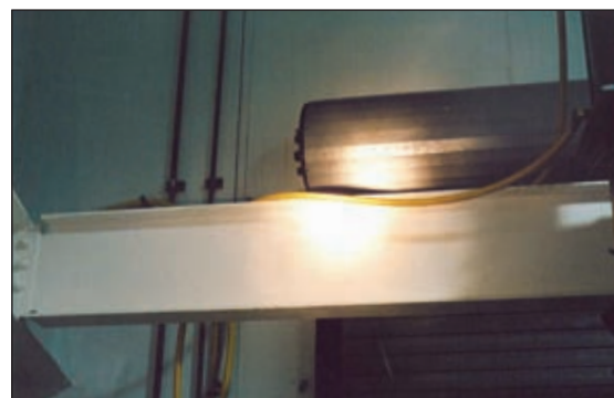
Fig. 2: Typical structural member coated with the acrylic elastomeric
