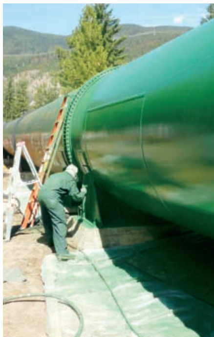
Fig. 12: Spray application of HRCSA finish coat
