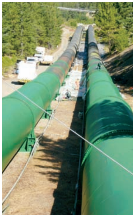
Fig. 13: Overview of coating work in progress
