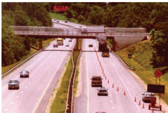
Fig. 1: Increasingly, bridge painting is done using mobile platforms with temporary lane closures. Courtesy of New Hampshire DOT
