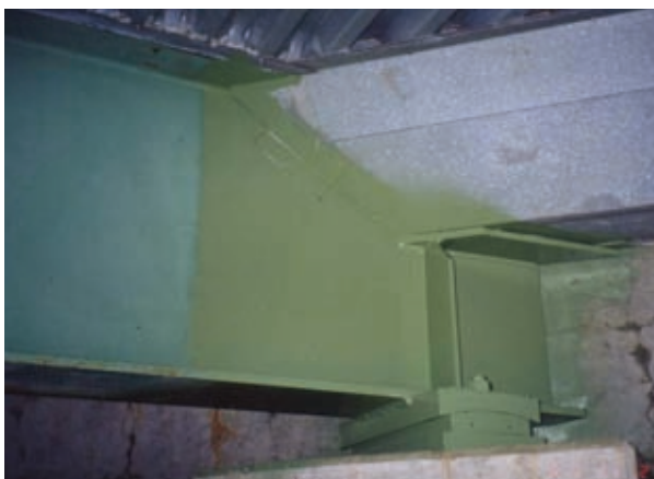
Fig. 4: Zone painting can focus resources on specific areas of the bridge threatened by relatively harsh micro-climates.
