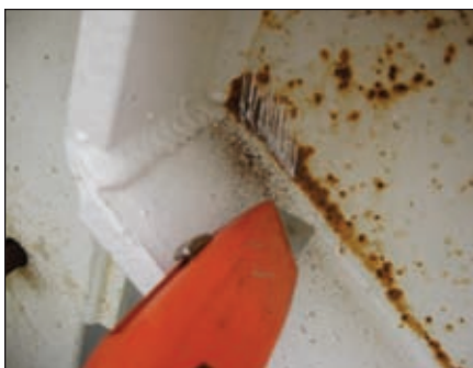
Fig. 5: Metallic residues from grinding operations collected in horizontal pockets that also collected water resulting in surface pinpoint rusting.
