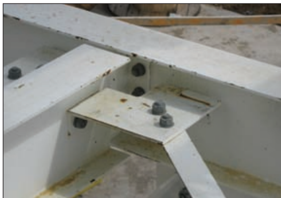
Fig. 1: Typical construction damage evident on exterior exposed steel components. Surface rust and dirt can be seen on the lower flange. Photos courtesy of the author
