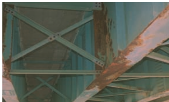
Fig. 2: Selective corrosion and paint failure under a leaking joint. Photo courtesy of the author
