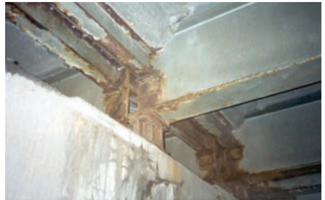
Fig. 3: It is common for a bridge to have significant deterioration directly underneath deck expansion joints, while the remainder of the structure is in relatively good condition. Courtesy of the author
