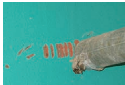
Fig. 3: Impact damage from earthquake
