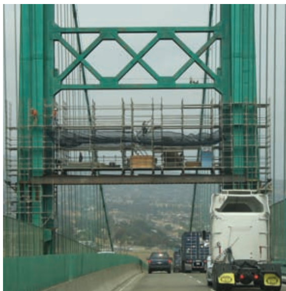
Fig. 1: Beams traversing roadway for upper tower scaffolding support
