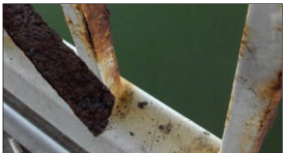
Patches of general corrosion on railing spindles, on the lower bridge sections
