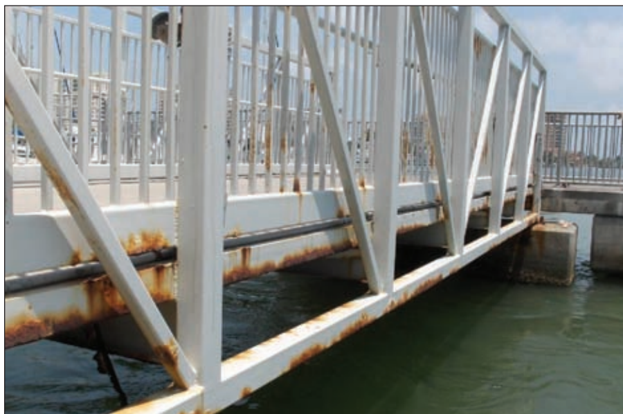
Pedestrian bridge showing extensive corrosion of the bridge components Photos courtesy of Richard Burgess
