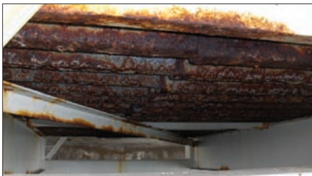
The galvanized deck pans beneath the center and north spans exhibited over 50% corrosion.
