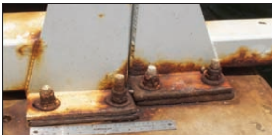
Corrosion on pier cap bearing and truss plate bolted connections
