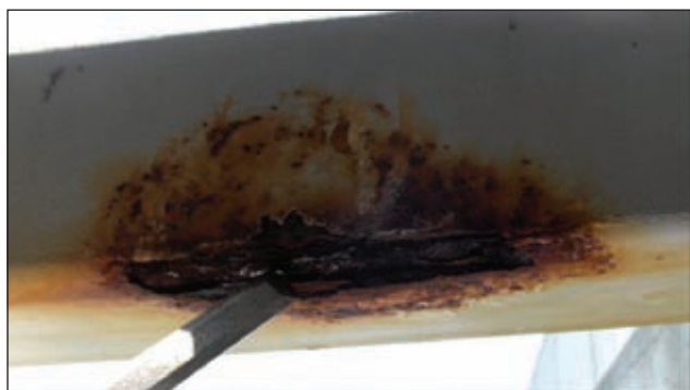
Undercutting of coating at areas of spot corrosion
