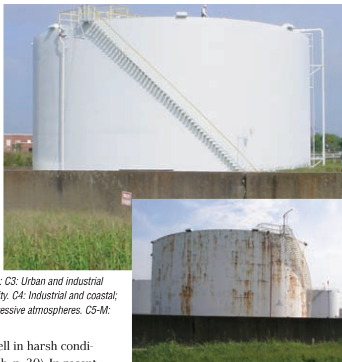
Fig. 4a (above): A tank coated with a single-component new generation waterborne latex containing "composite particles." 4b (below): The tank before overcoating. Courtesy of Dow Coating Materials (formerly Rohm & Haas Company)
