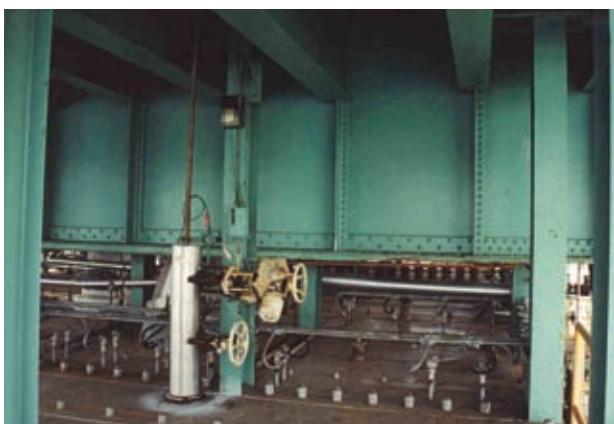
Fig. 5a (above): Thermal generation plant (fueled by natural gas). Steel overated with an acrylic latex. 5b (below): The coating 15 years later, maintenance free, at same location: the structure is open to a seacoast environment. Courtesy of Frank Bird, Glidden Paints and Peter Roberts, Devco Coatings
