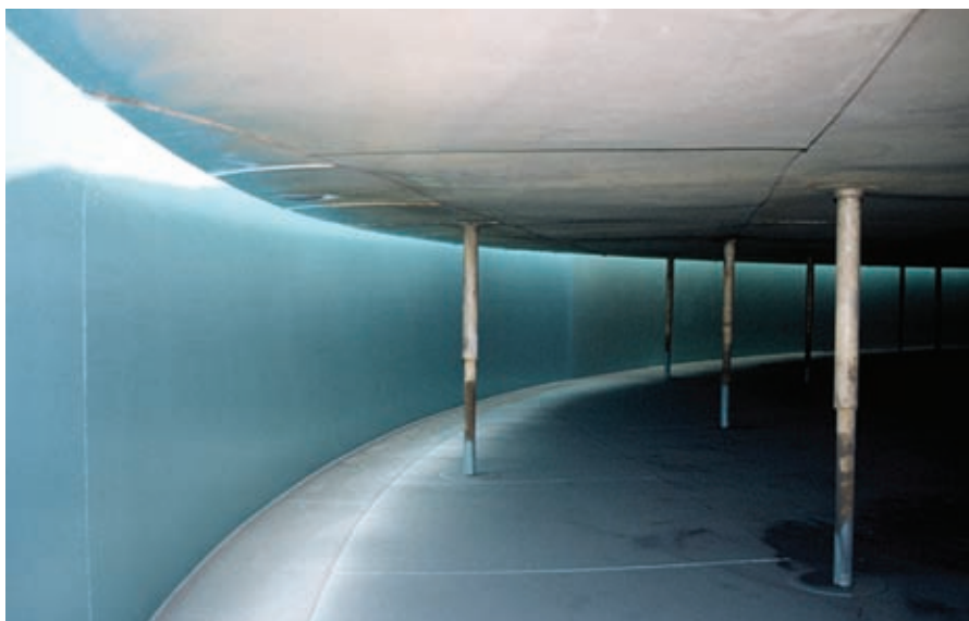
Fig. 8: One-coat solvent-free advanced hybrid epoxy in crude oil storage tank. Courtesy of Darryl Corbin, Enviroline, High Performance Coatings and Linings
