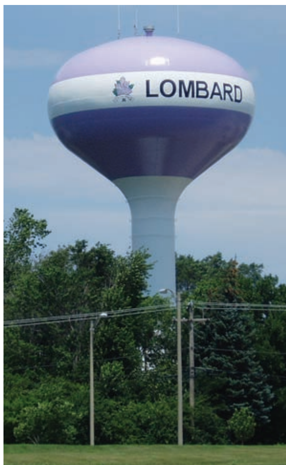
This tank in Lombard, IL, "The Lilac Village," is still a community landmark three years after the tank was recoated with a fluorourethane coating system.
