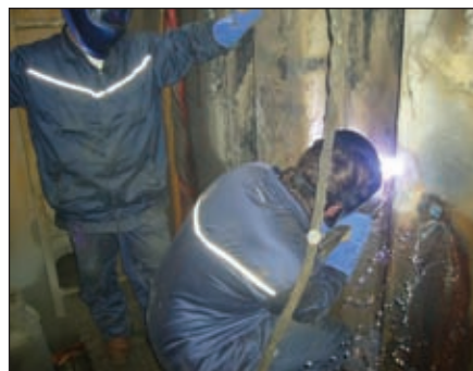
Fig. 5: Welding new steel plates over holes in the steel and over steel less than 5 mm thick
