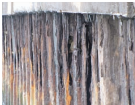
Fig. 1: The USACE knew little about the condition of the steel underwater at the U.S. Naha military port on Okinawa until the area was dewatered Photos courtesy of the author
