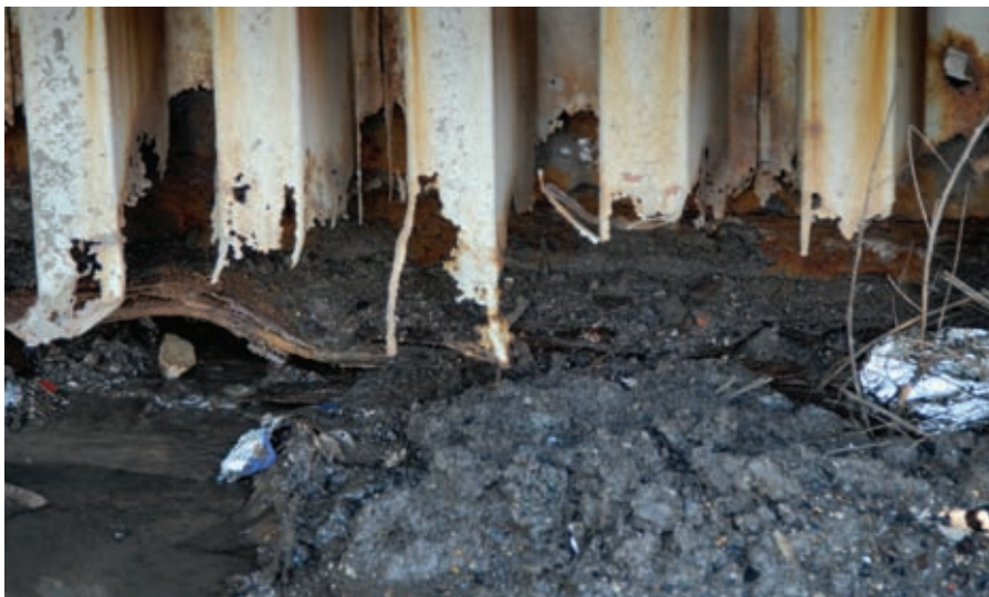
Corroded pile revealed during levee inspection. Courtesy of the U.S. Army Corps of Engineers
