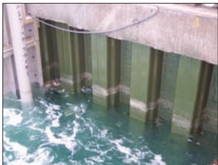
Fig. 6: The coating can cure underwater at relatively low temperatures.
