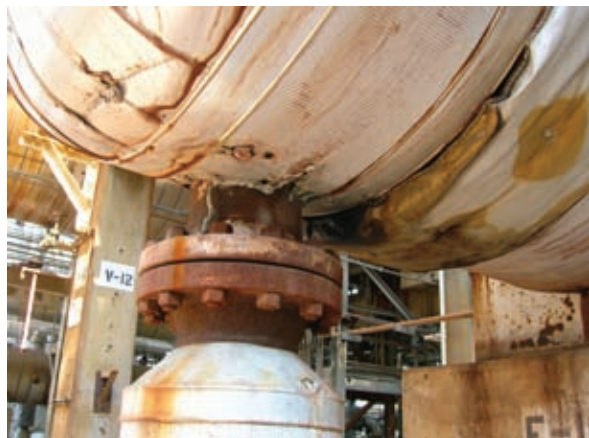
Fig. 1: Corroded sheet metal cladding, soaked-through insulating blanket, and extensive rust on the exposed flange indicate potential problems under the insulation.
