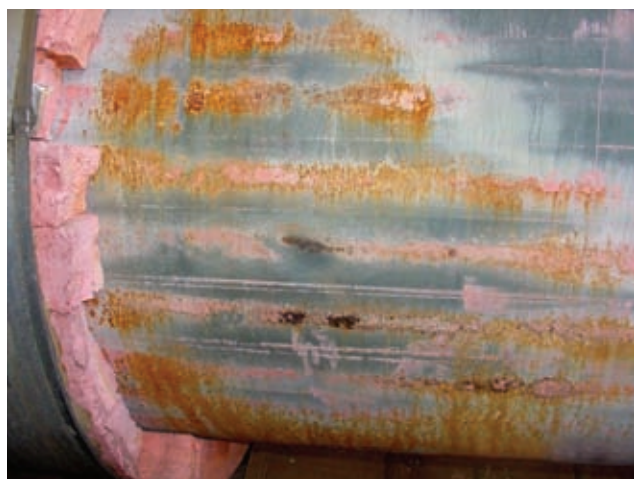
Fig. 3: Partially failing but repairable 20-year-old inorganic zinc coating with calcium silicate insulation removed.
