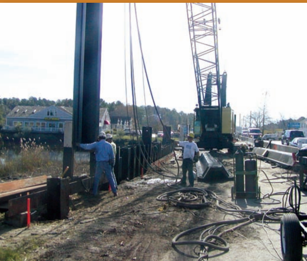
Driving piles coated with CTE Courtesy of the U.S. Army Corps of Engineers
