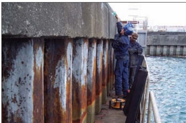
Fig. 4: Filling holes and voids with polyurethane foam and remodeling the surface with special cement
