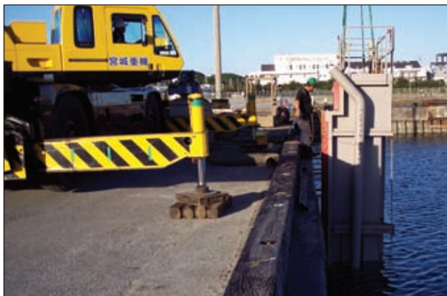
Fig. 2: Modular cofferdam that was shipped in containers to the site and installed for work at the bulkhead.
