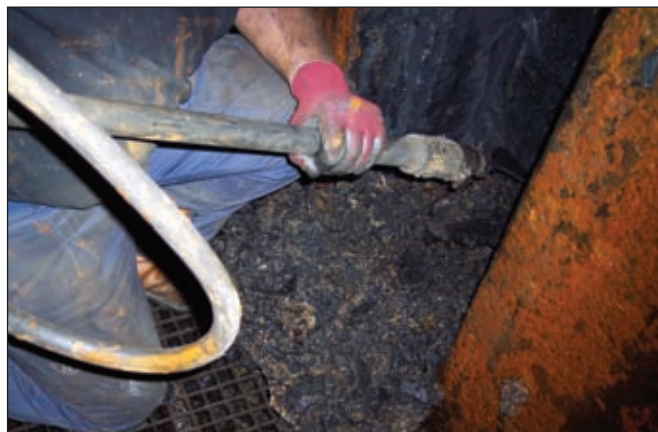
Fig. 3: After the initial cleanup process, virtually all loosely adhered material was removed.
