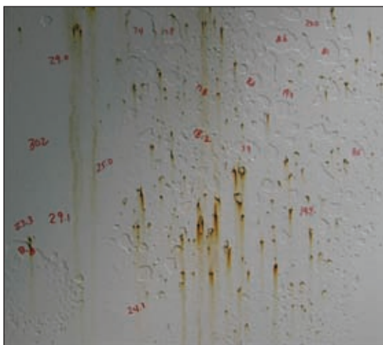
Fig. 2: Premature rusting of lining system
